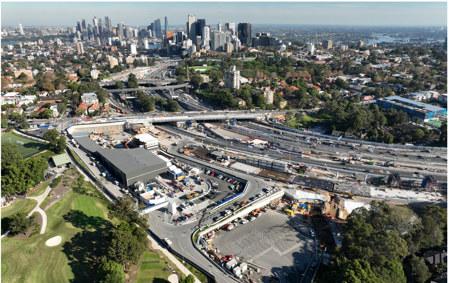
Cammeray construction site, Cammeray.
