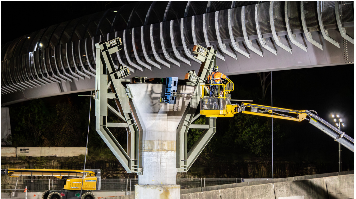
The new Falcon Street shared user bridge girder installation.
