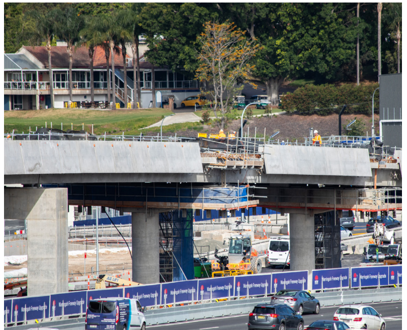
The new Miller Street southbound on ramp.
