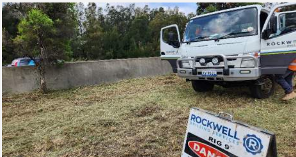
Photo 1: 28/02/2024: Representative image of site location (BH98A) - Pile
