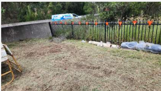
Photo 5: 28/02/2024: Representative image of site location (BH98A) - Pile
