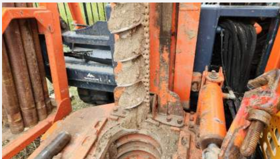
Photo 24: 27/02/2024: Representative image of soil material (BH99A) - Pile
