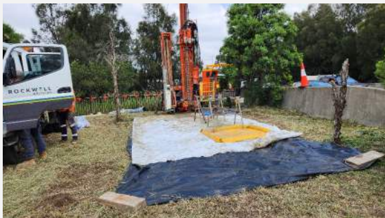
Photo 3: 28/02/2024: Representative image of site location (BH98A) - Pile
