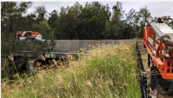
Photo 18: 27/02/2024: Representative image of site location (BH99A) - Pile
