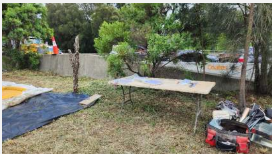
Photo 4: 28/02/2024: Representative image of site location (BH98A) - Pile
