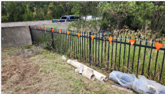
Photo 7: 28/02/2024: Representative image of site location (BH98A) - Pile
