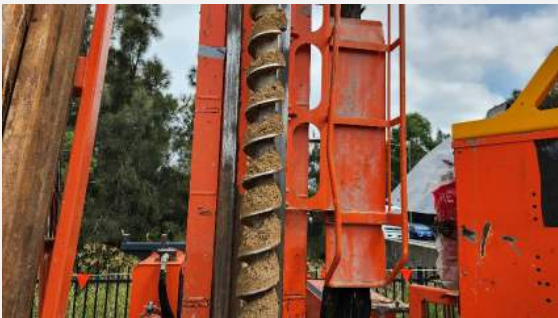
Photo 13: 28/02/2024: Representative image of soil material (BH98A) - Pile
