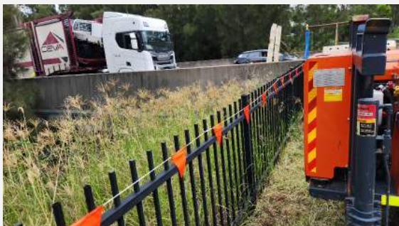
Photo 6: 28/02/2024: Representative image of site location (BH98A) - Pile
