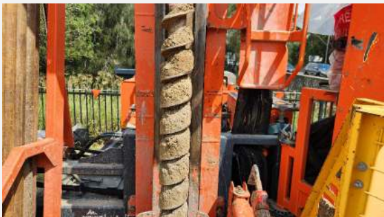
Photo 12: 28/02/2024: Representative image of soil material (BH98A) - Pile
