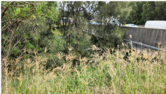
Photo 9: 28/02/2024: Representative image of site location (BH98A) - Pile
