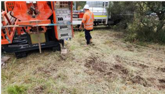
Photo 20: 27/02/2024: Representative image of site location (BH99A) - Pile
