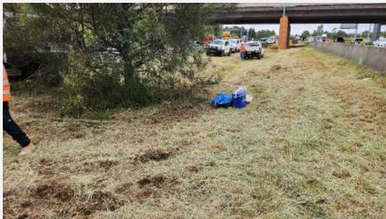
Photo 19: 27/02/2024: Representative image of site location (BH99A) - Pile
