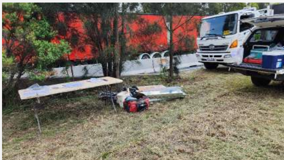
Photo 2: 28/02/2024: Representative image of site location (BH98A) - Pile
