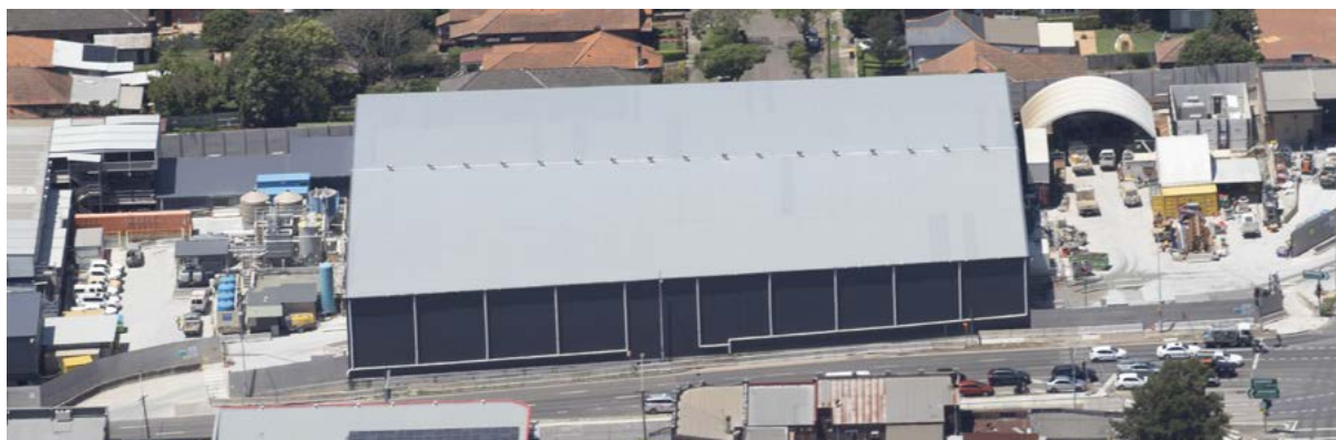
Acoustic sheds are designed to minimise noise, light and dust spill on the local community and are commonly used on tunnelling projects. Photo: example acoustic shed.
