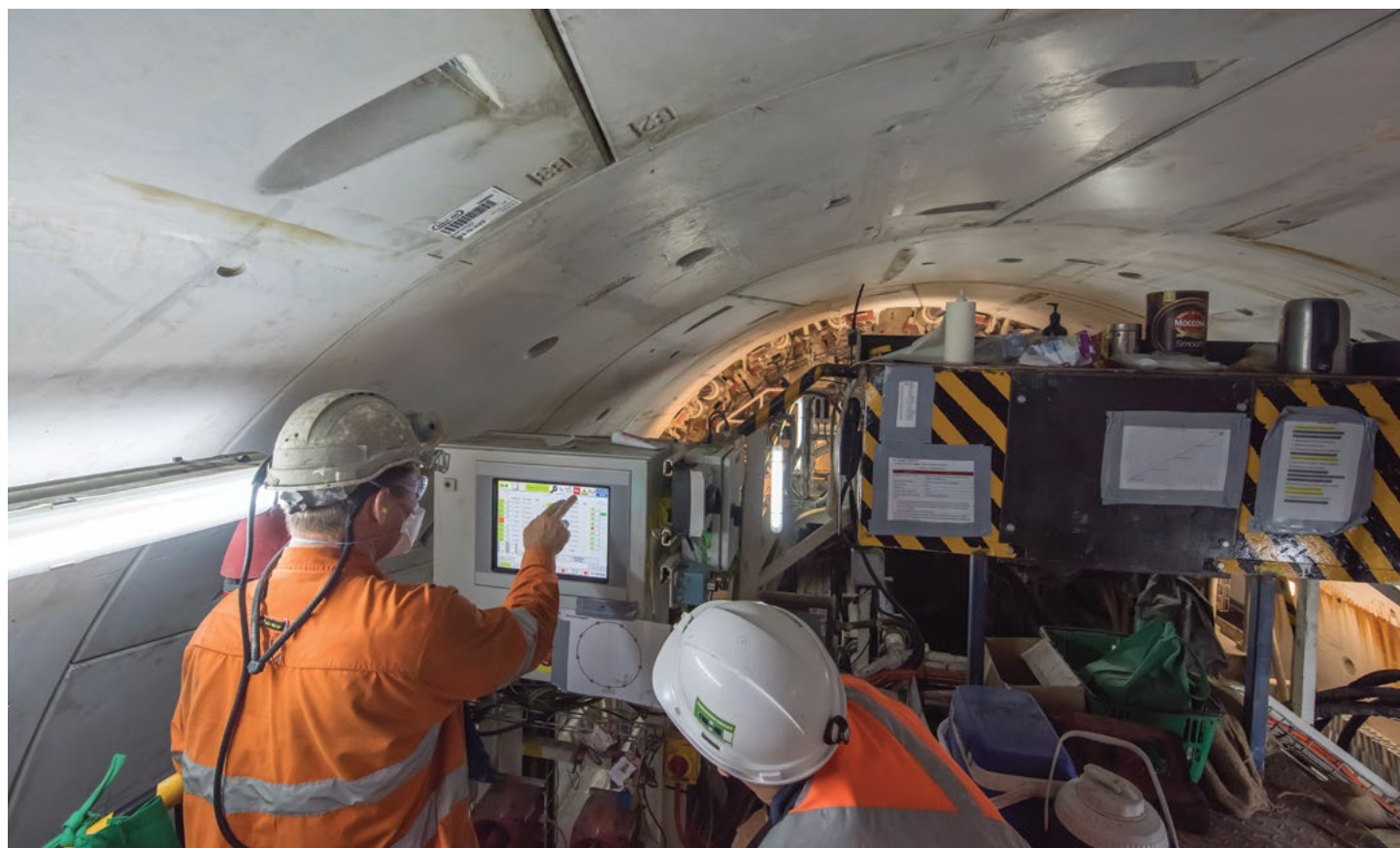
Inside a tunnel boring machine (TBM).
