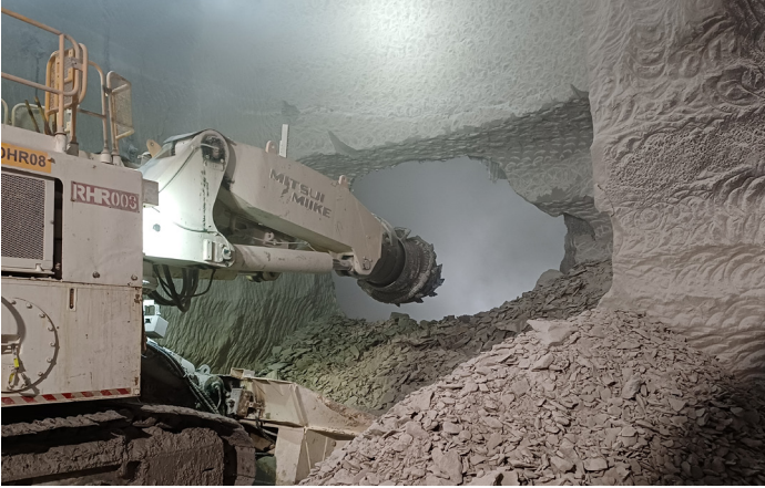
Roadheader breaking through from Rockdale to Arncliffe, August 2024
