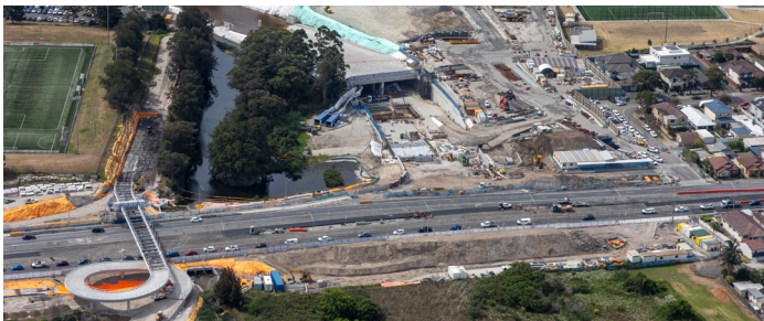
President Avenue and Bicentennial Park tunnel portal, September 2024
