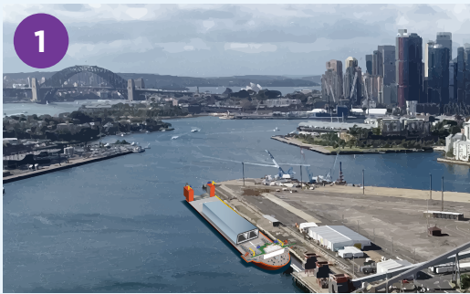
1 Construction and fitout of immersed tube tunnel units at White Bay
