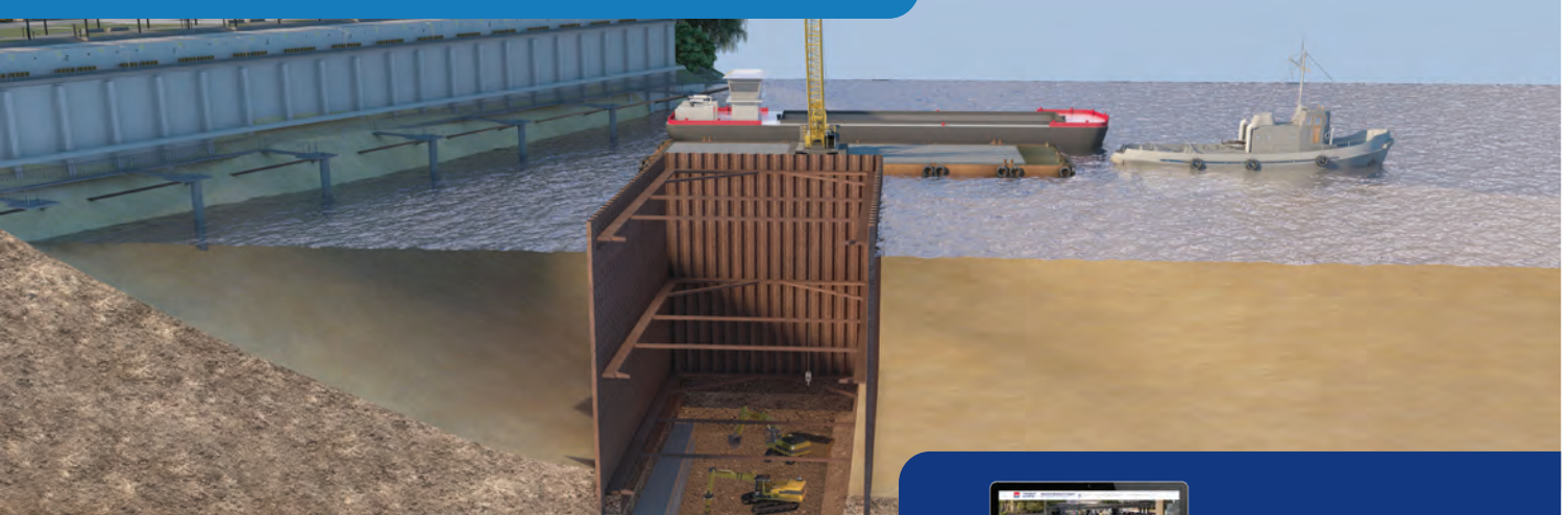
Artist's impression of cofferdam construction in Sydney Harbour
