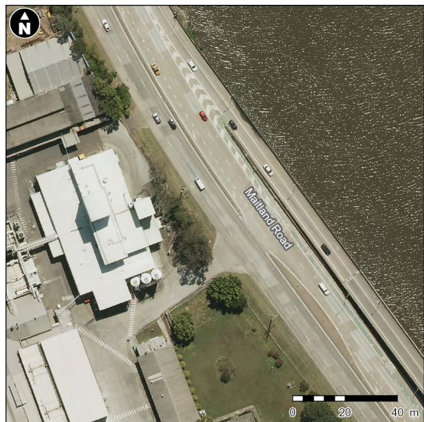
Plate 2.17 Intersection of Brancourts access road and Maitland Road
