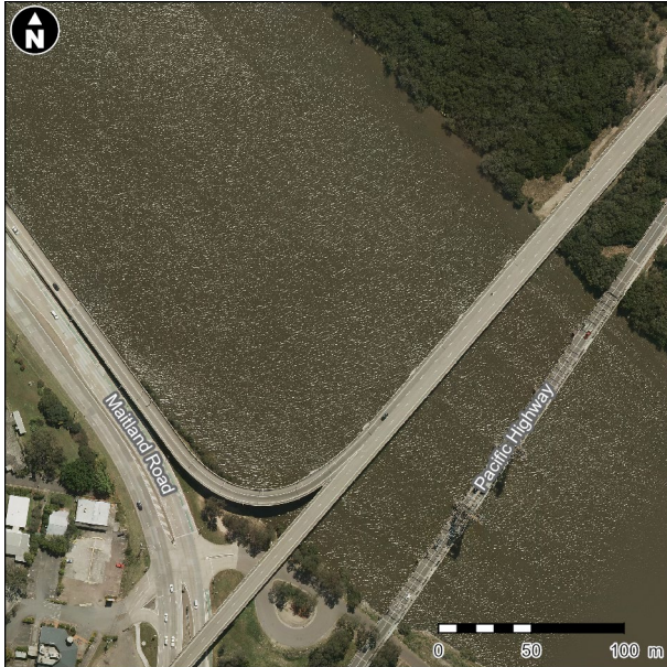
Plate 2.13 The A1 Pacific Highway south-eastbound entrance ramp and three lane northbound bridge over the Hunter River.
