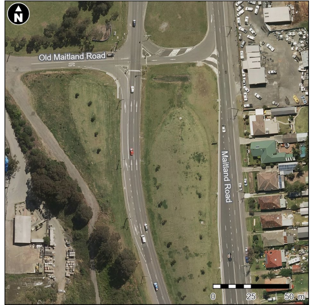
Plate 2.2 Northbound approach to Old Maitland Road Sandgate and Maitland Road intersection
