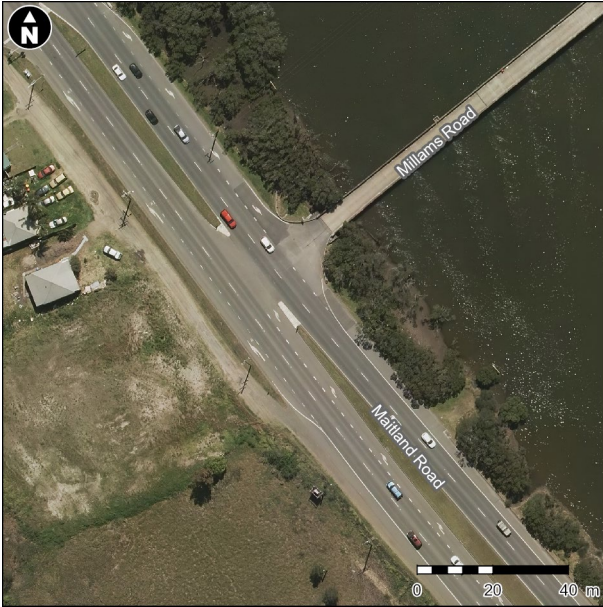
Plate 2.5 Millams Road and Maitland Road intersection
