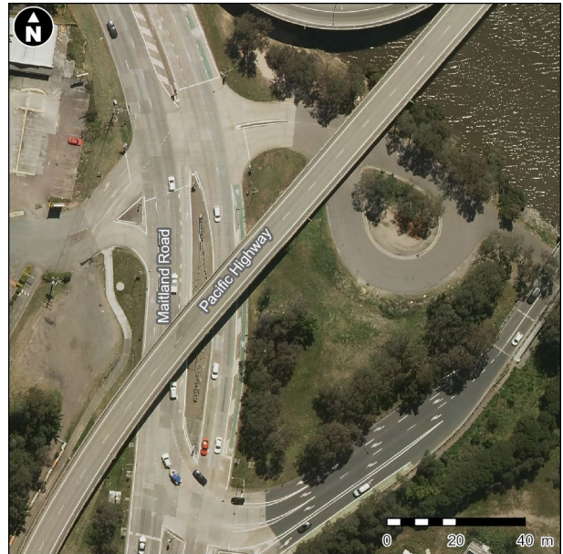
Plate 2.12 Intersection of Maitland Road and a U-turn around facility underneath the northbound entrance ramp of the A1 Pacific Highway to the right and the southern access road to the Oak Factory and Maitland Road to the left of the image
