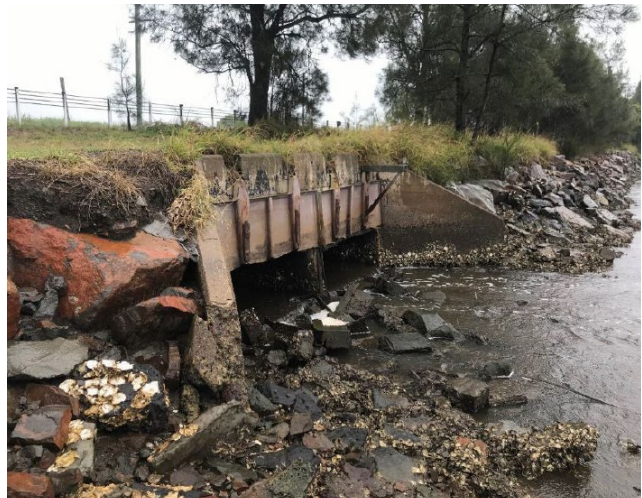
Plate 2.19 Reinforced concrete box culvert 02, drainage system 24
