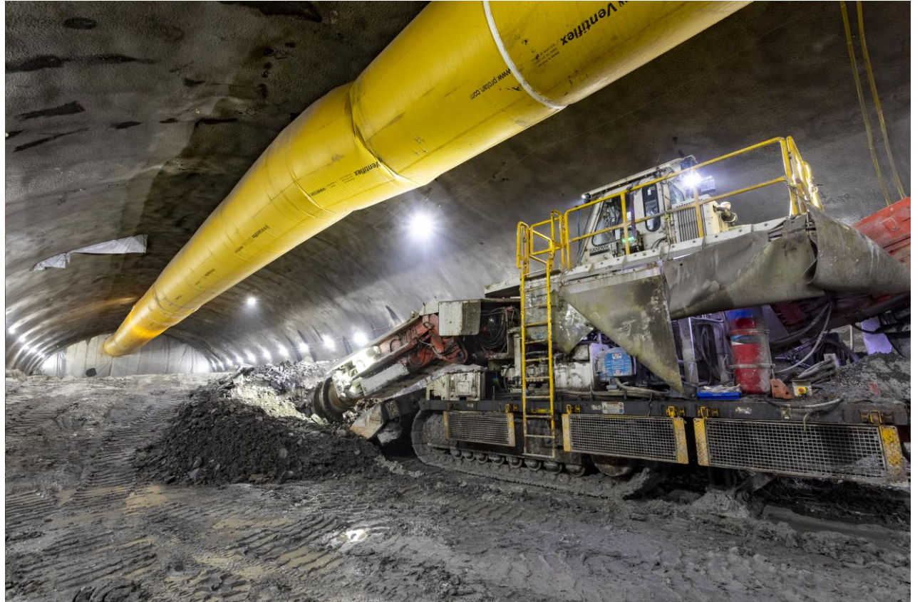
Image of a roadheader in operation.
