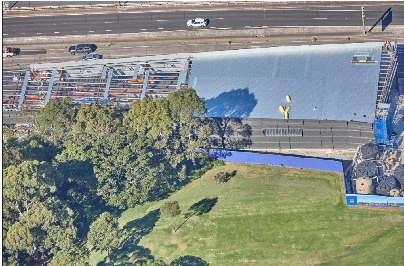
Ridge Street acoustic shed under construction in April 2024.
