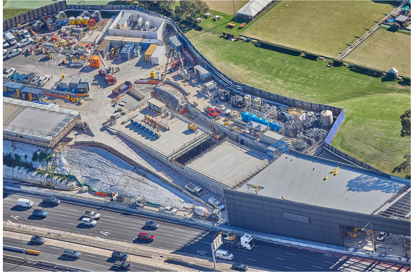
Aerial view of the off ramp portal at Ridge Street.
