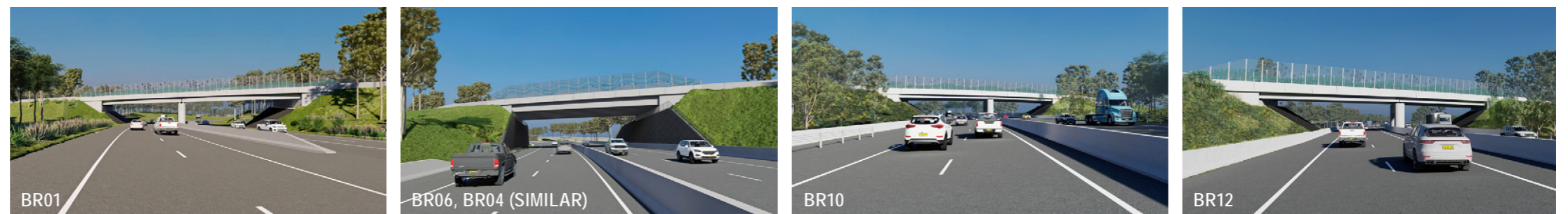
Figure 61: M1 Pacific Motorway Extension to Raymond Terrace - northern and southern packages integration
