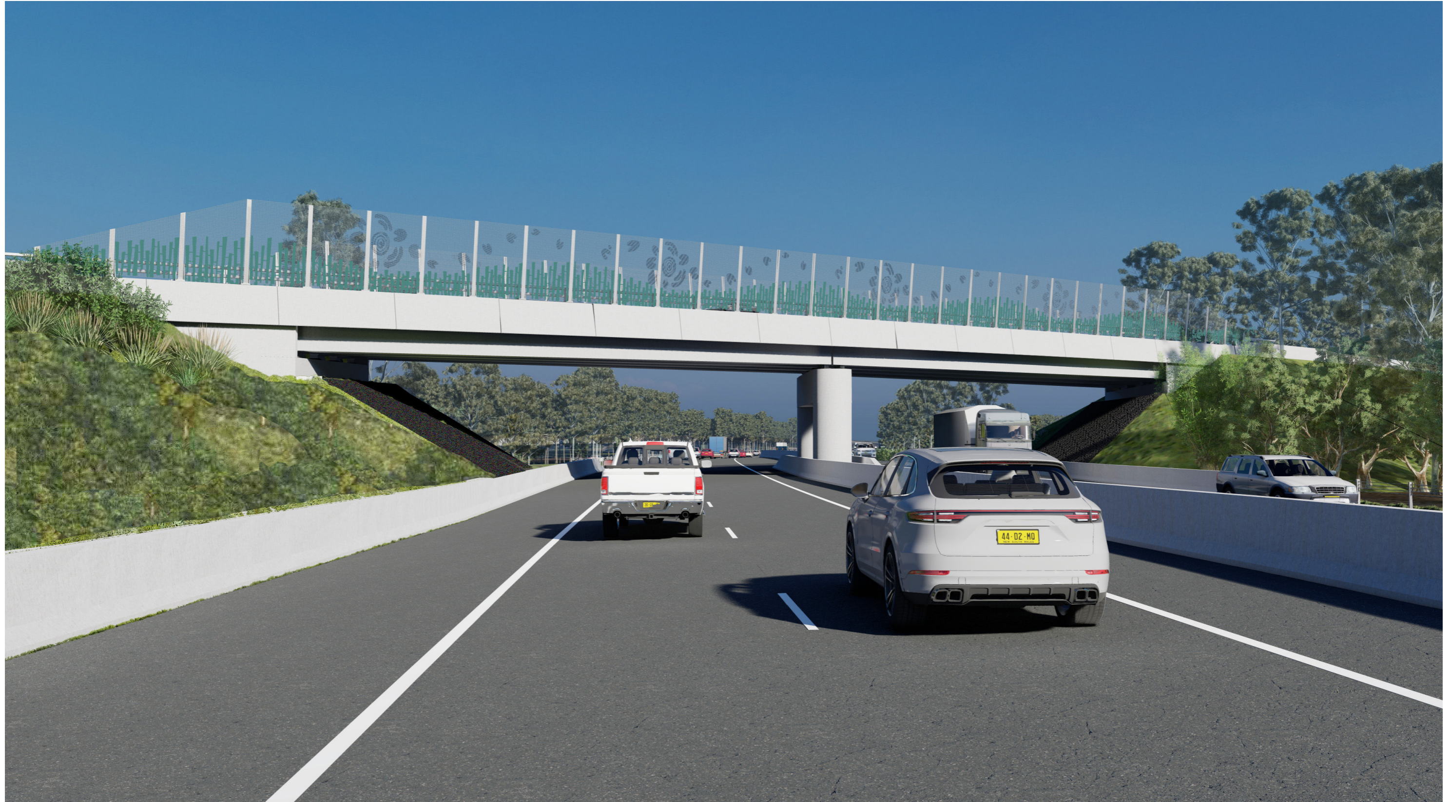
Figure 47: BR12, looking north
