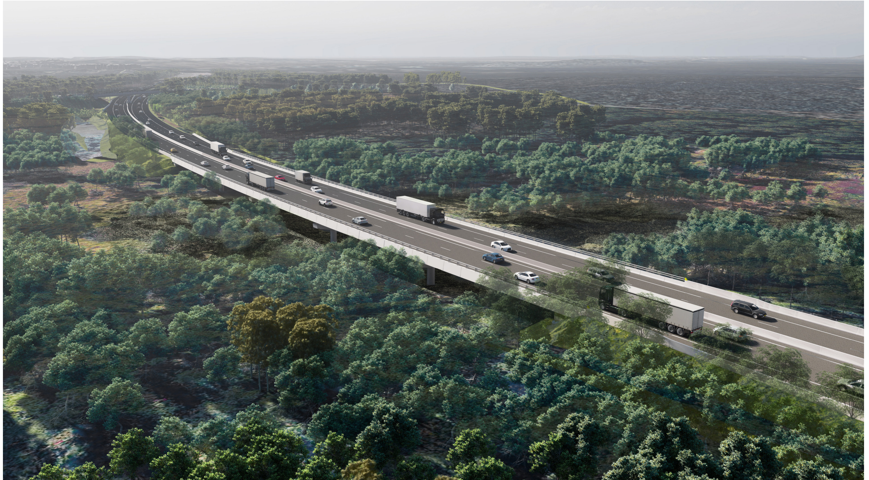
Figure 42: BR11 - aerial view, looking north
