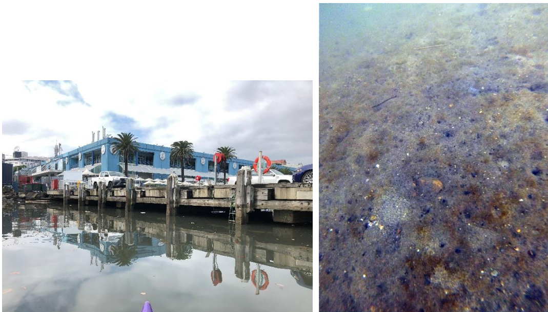
Left – Concrete Wharf requiring two protection piles for relocation of the net spooling berth; right – typical sediment for new piles (bare silty sand with fine filamentous algae crust)
