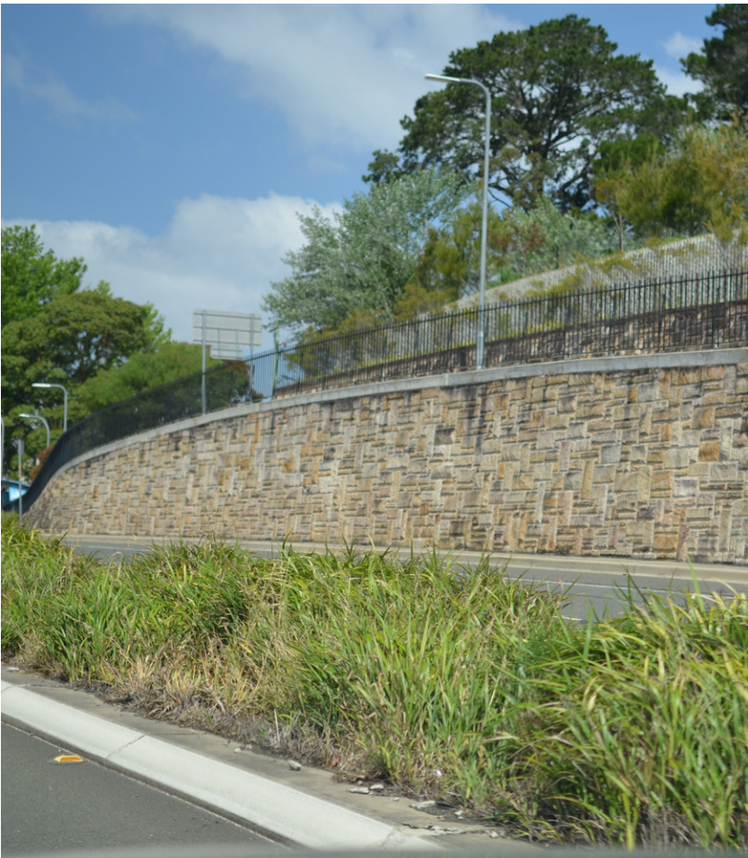
Figure 4-9 Type 1 - High quality finishes and slight incline used in highly visible settings along the Great Western Highway at Lawson
