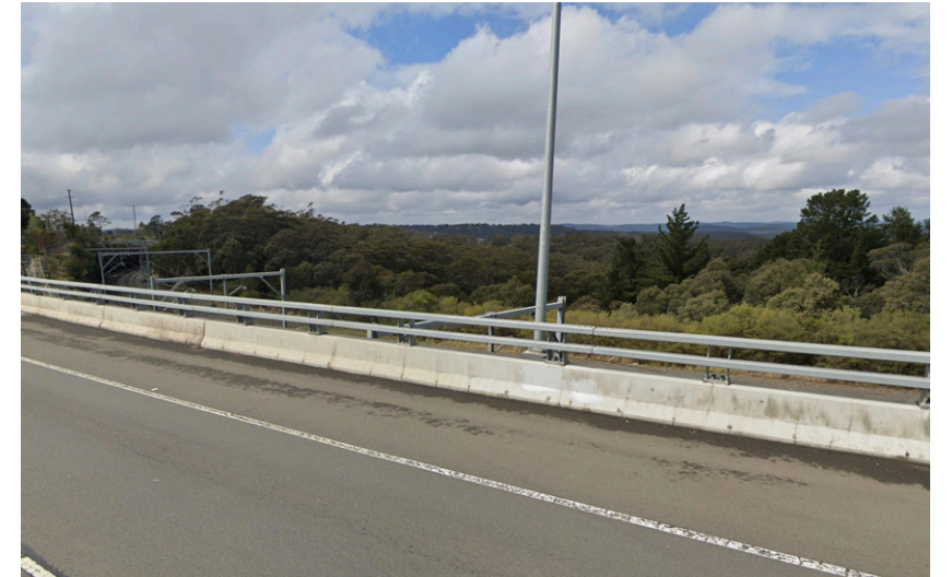
Figure 4-12 F-Type Barriers with rails enable views to permeate through to views beyond (Lawson) Source: Google Street View
