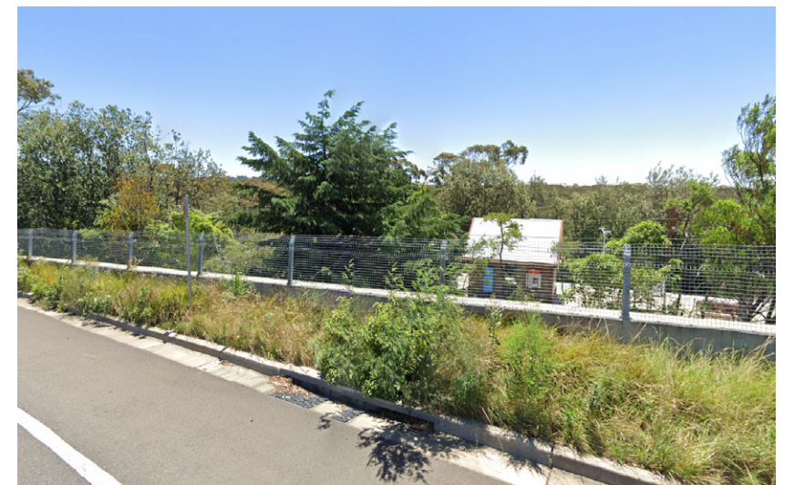
Figure 4-13 F-Type Barriers with fencing atop to restrict access into the rail corridor (Bullaburra) Source: Google Street View
