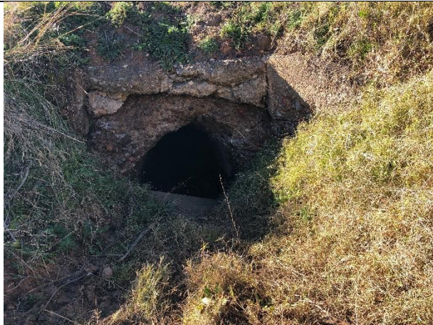
Plate 19: View east at culvert 2 (1.3 kilometres from bridge) (photo AECOM)
