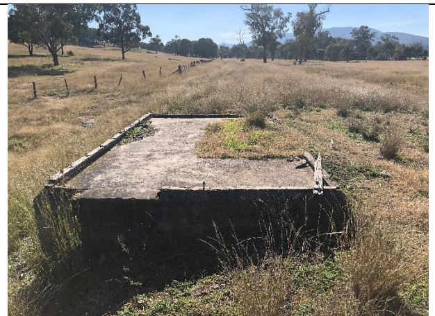
Plate 14: View north at concrete base (photo AECOM)
