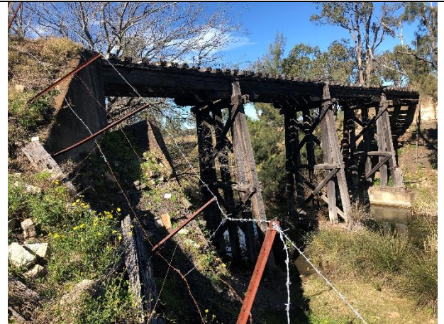
Plate 12: View south-east towards bridge (photo AECOM)
