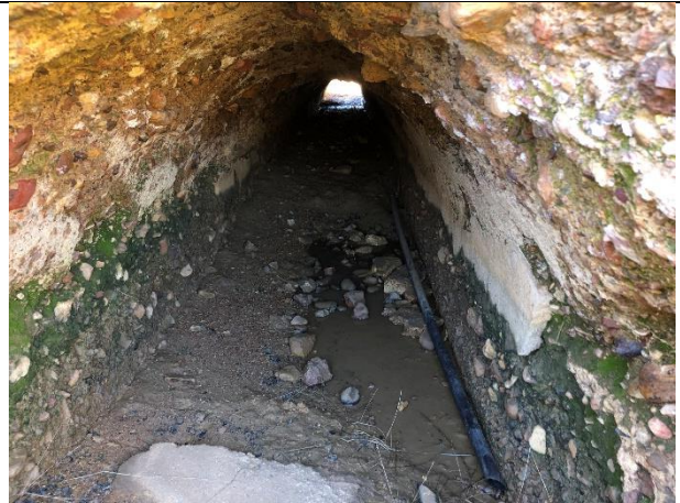
Plate 20: View through culvert 2 (1.3 kilometres from bridge) (photo AECOM)
