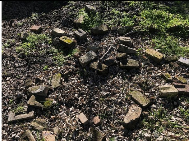
Plate 15: Rubble beneath bridge (photo AECOM)
