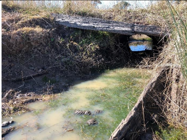
Plate 17: View east at culvert 1 (850 metres north of bridge) (photo AECOM)
