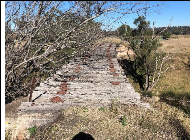
Plate 11: View south across bridge (photo AECOM)
