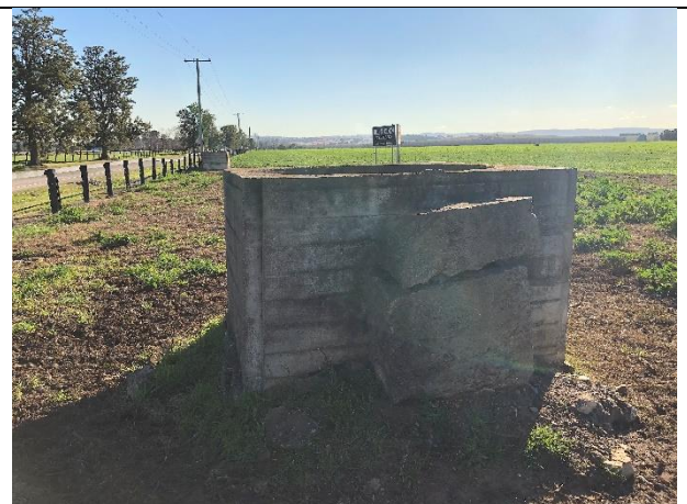
Plate 2: Concrete tank (photo AECOM)
