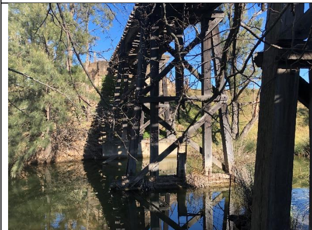
Plate 13: View south from beneath bridge (photo AECOM)
