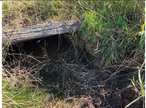
Plate 18: View west at culvert 1 (850 metres north of bridge) (photo AECOM)
