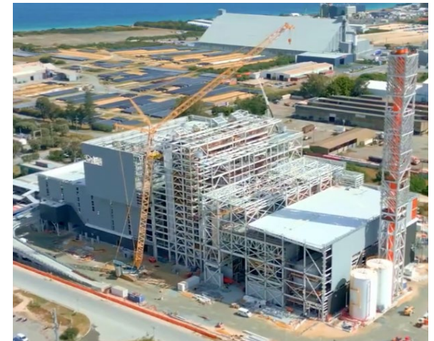
Kwinana Waste to Energy, Perth
