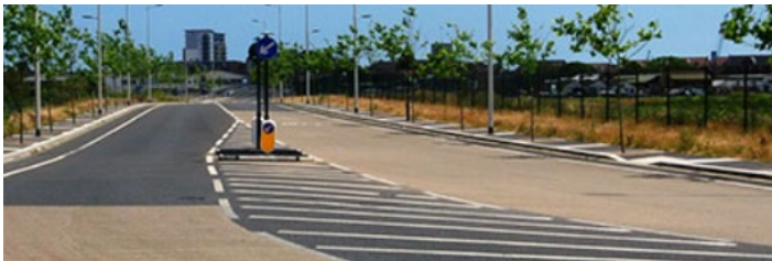
30,000t IBAA used for road construction and embankment (UK)
