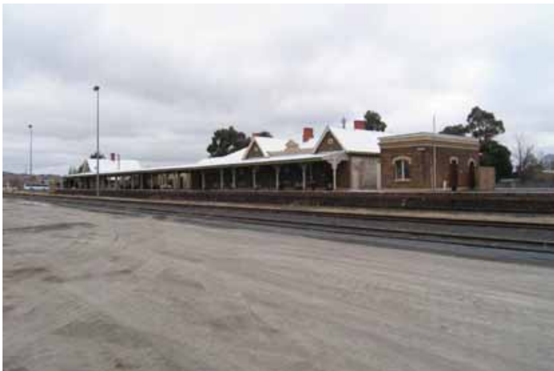
Plate L3-2. Blayney Railway Station buildings, Blayney, looking south-east.
