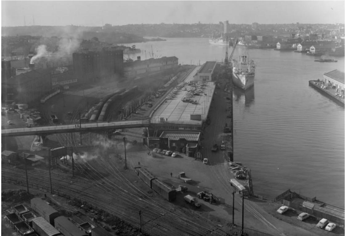
Figure 7-8 The industrial waterfront around the promontory at Pymont
