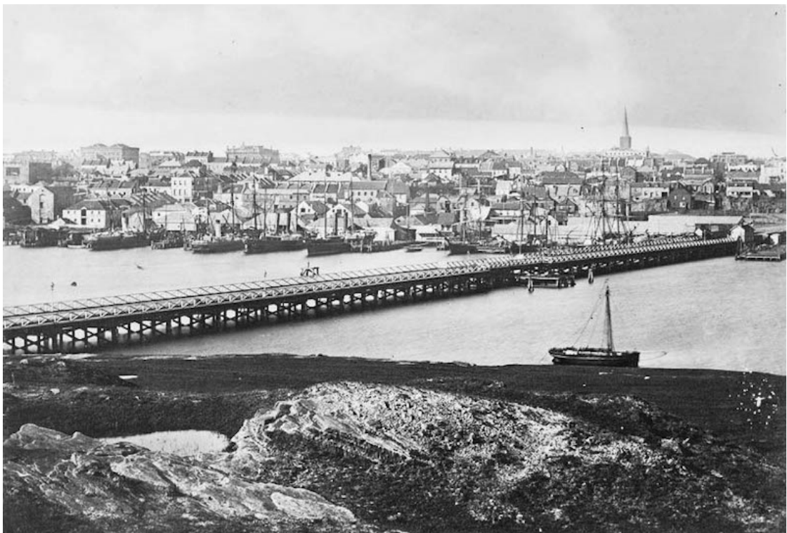
Figure 7-5 Extract of an image at the Pymont bridge 1874
