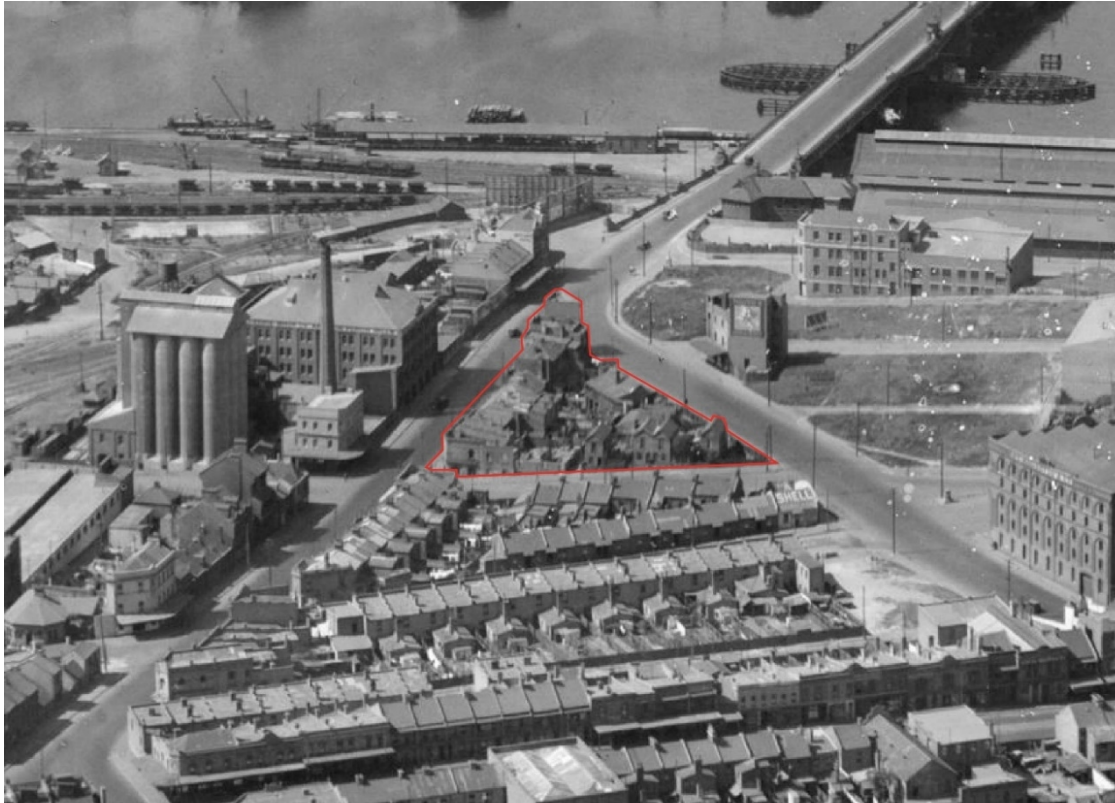
Figure 7-10 Extract from Milton Kent aerial photos. Terrace Housing and Shops located on Union Street, ca. 1920-1930. Portion of the site indicated in red
