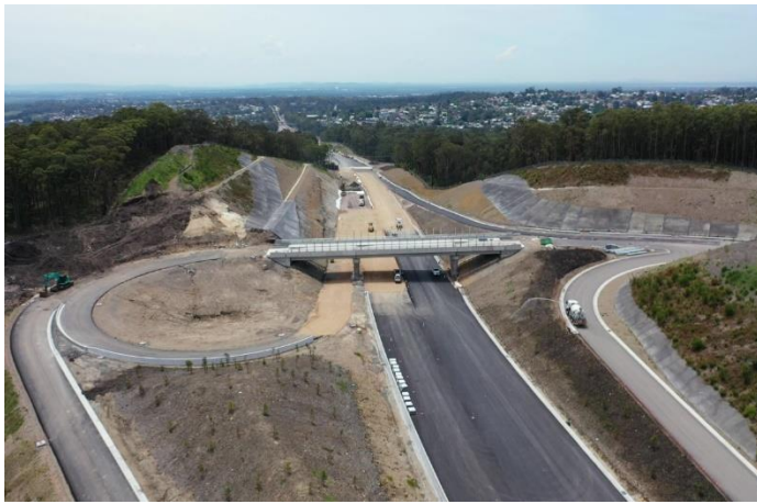
Hospital interchange with Super T girder bridge, October 2025
