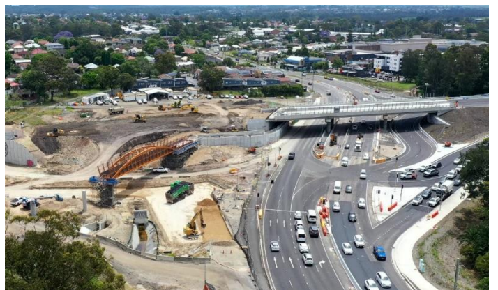
Northern interchange looking west, showing new steel arch pedestrian and cyclist bridge, November 2025
