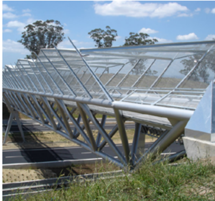
Existing M7 cycleway bridge
