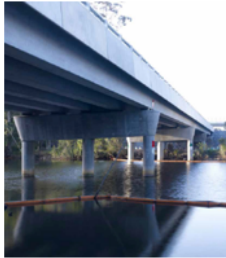
Bonville Upgrade creek bridge
