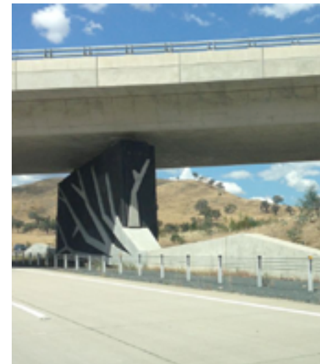
Voided slab - Wagga Wagga overpass
