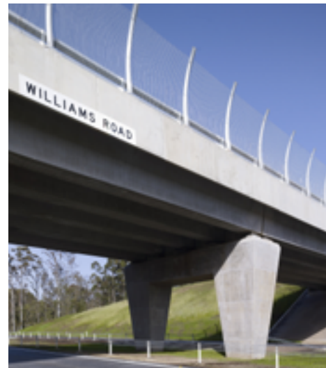
Portal frame structure pier - Bonville Bypass
