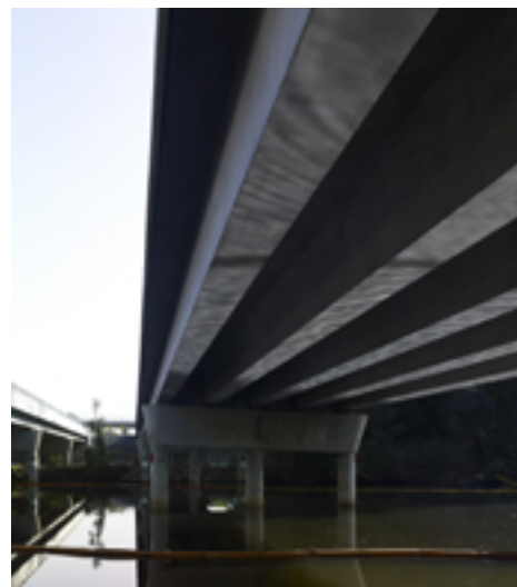
Super-T girder - Bonville Bypass
