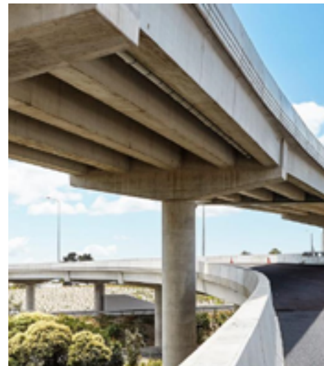
Circular piers with articulated capital
