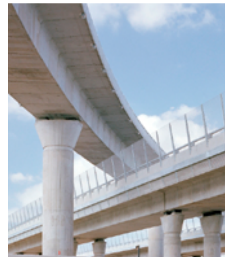
Box girder - M7 Motorway
