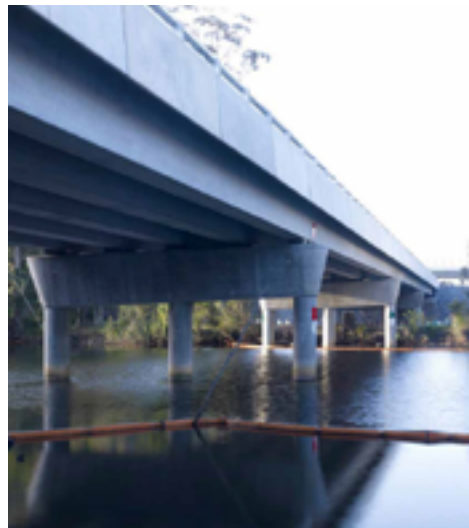
Circular piers with headstock - Bonville Bypass
