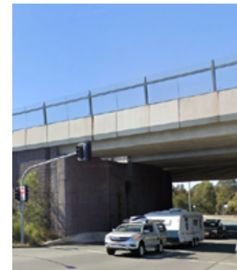
Walled abutment - Banora Point Upgrade
