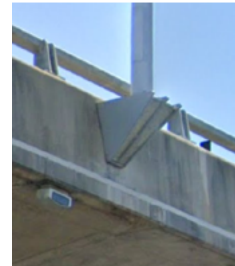
Existing M7 Motorway lighting corbel
