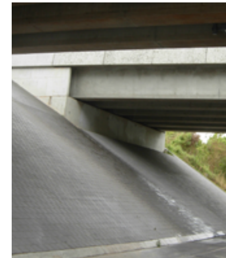
Spill through abutment
