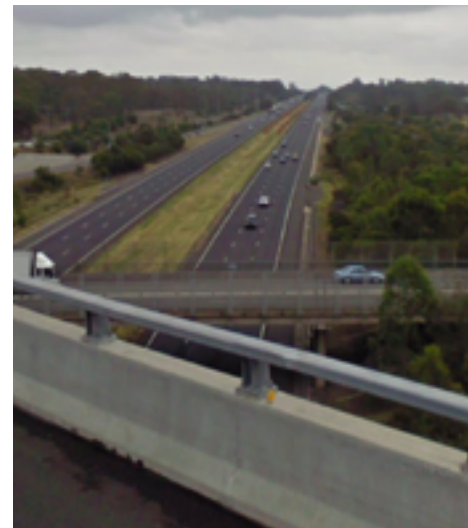
M7 Motorway - Single rail barrier
