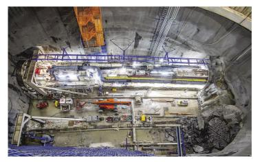
TBM Peggy breaking through at the Airport Terminal temporary shaft while TBM Eileen is traversing the shaft.
