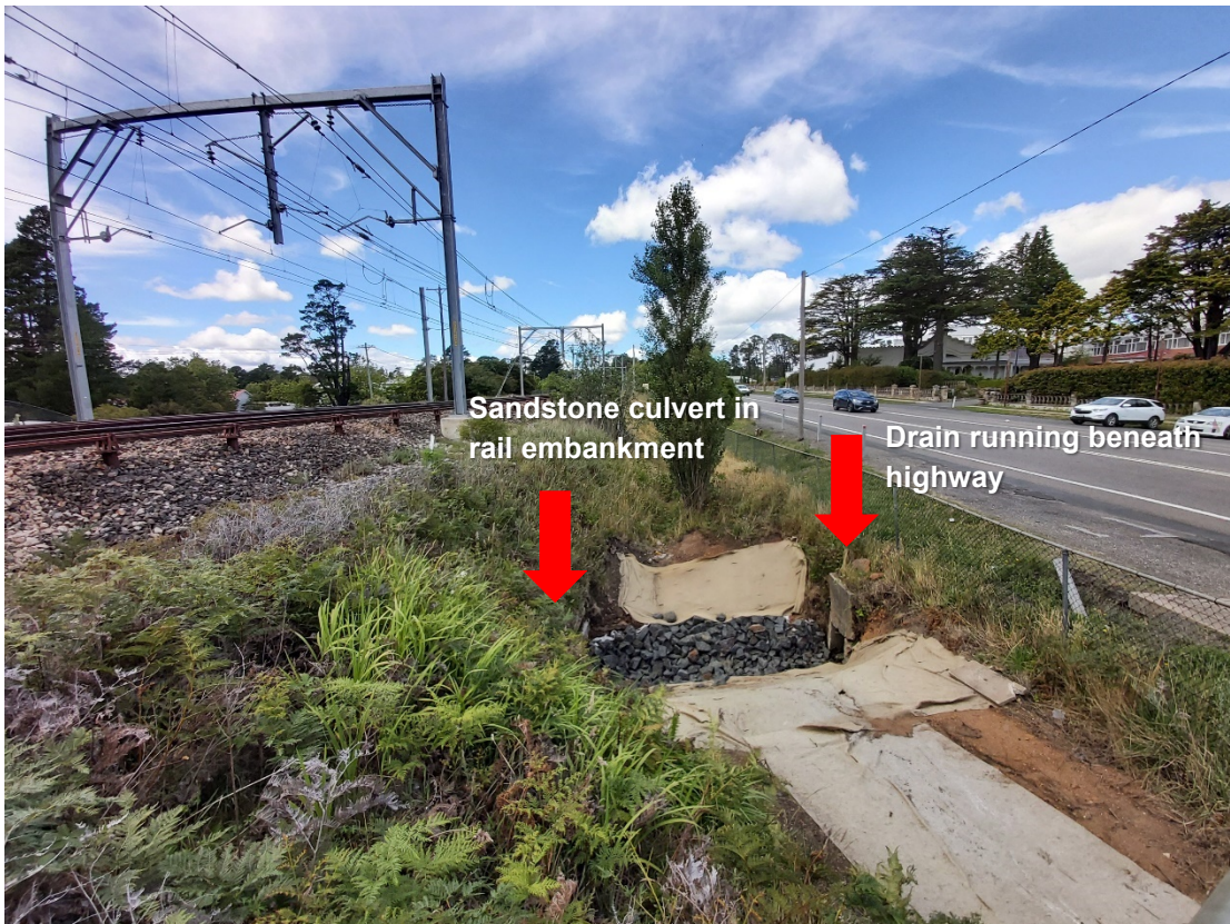
Plate 4.74: Sandstone culvert on western side of railway embankment showing proximity to Great Western Highway and drain running beneath highway (right), looking south (RPS 2020)
