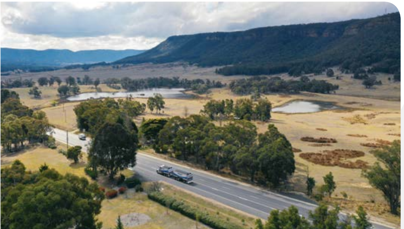
Great Western Highway looking towards Hartley Valley
