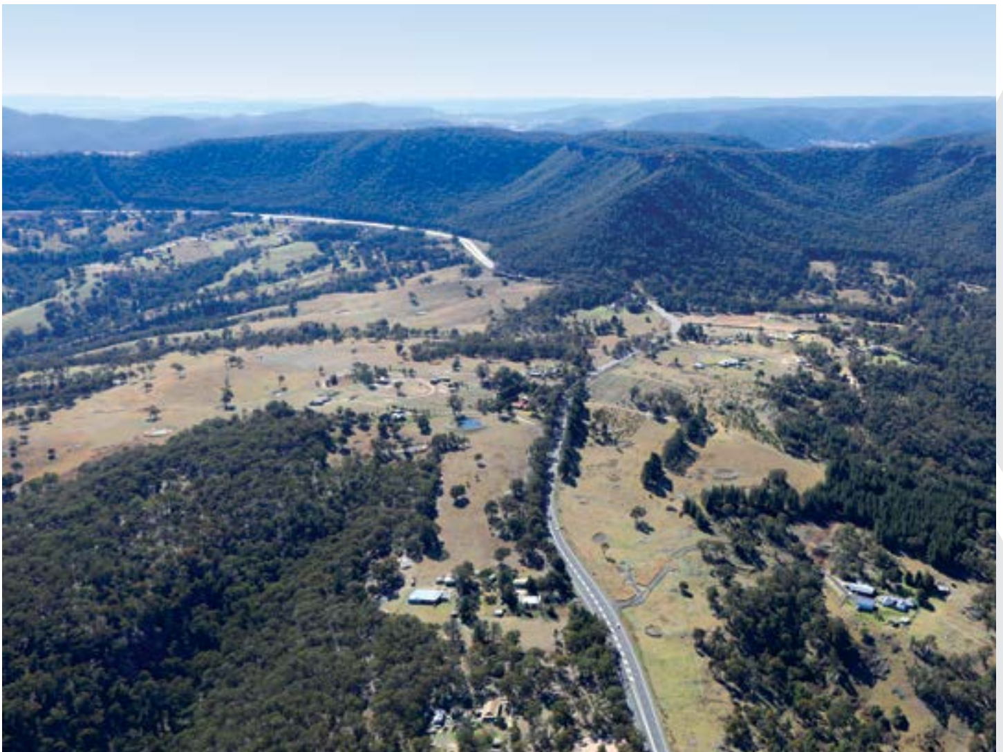
Great Western Highway looking towards Hassans Walls
