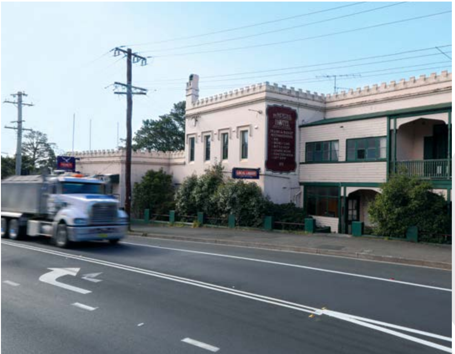
Great Western Highway at Mount Victoria
