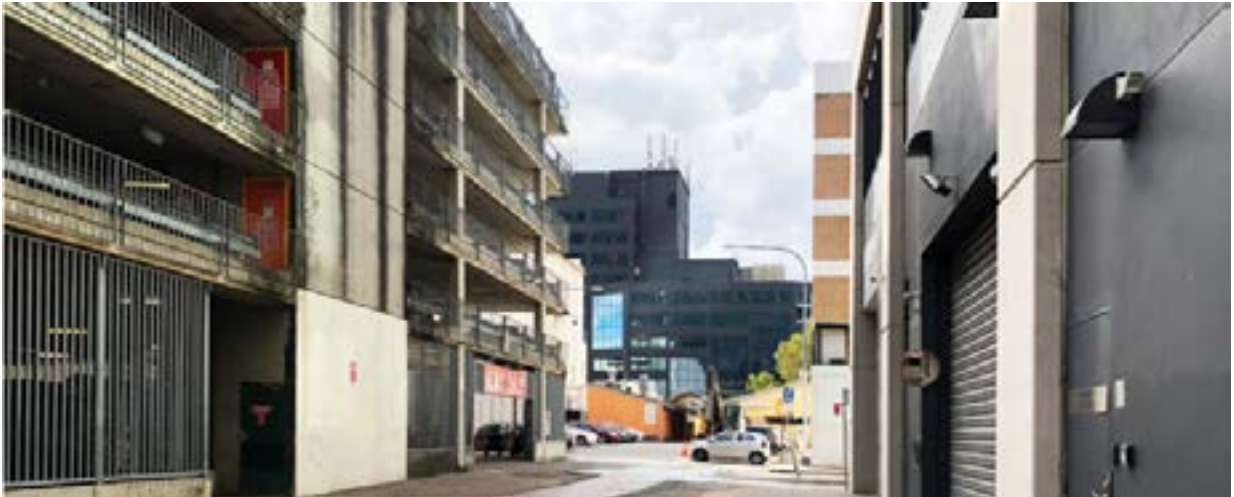
Figure 2-6 Looking north from the City Centre Car Park
