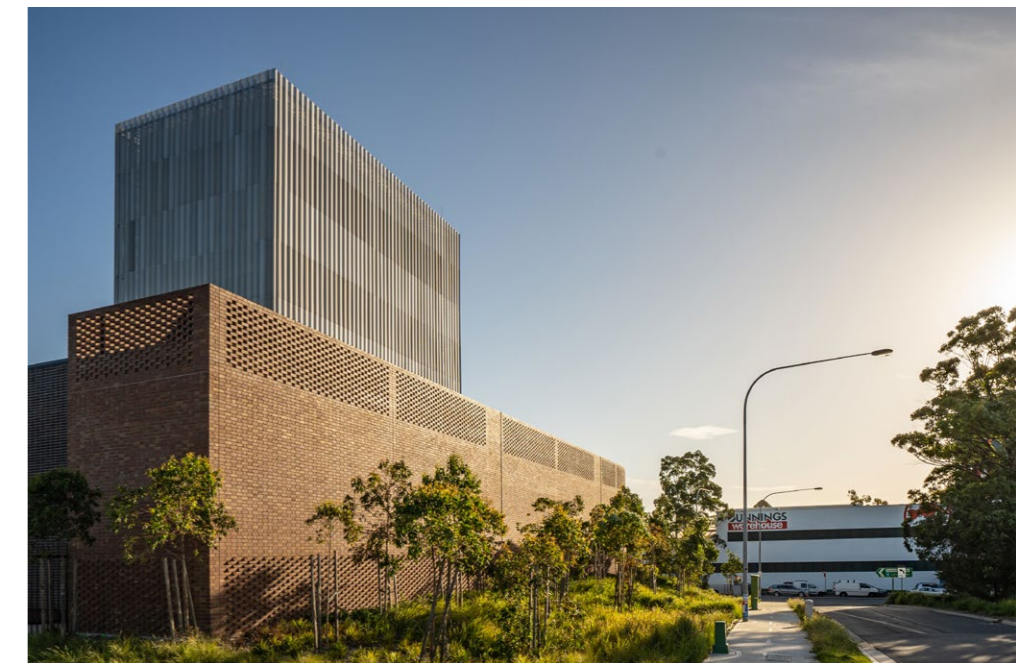
Figure 47: M4 East ventilation building, Haberfield
