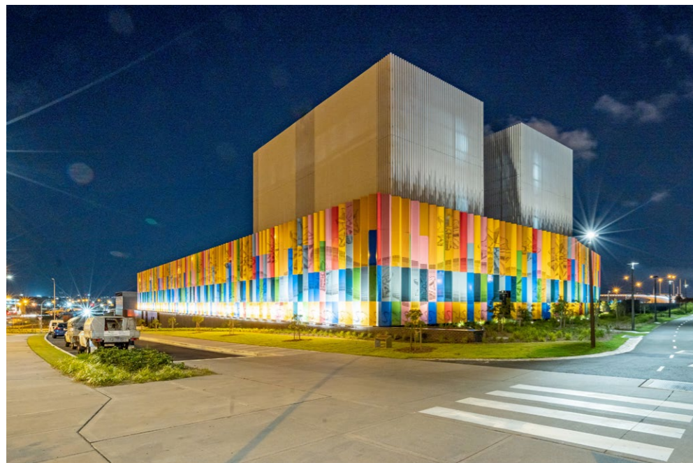
Figure 45: St Peters Interchange ventilation building, Sydney
