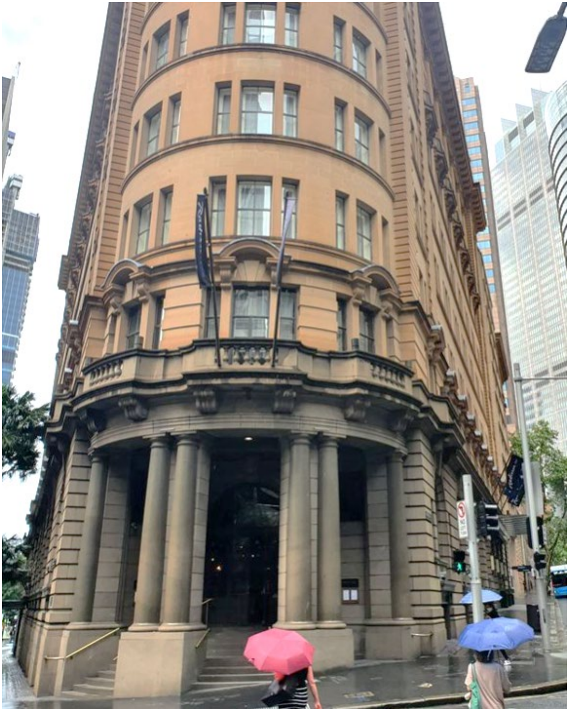
Figure 2-17 Radisson Blu Plaza Hotel at 27 O'Connell Street
