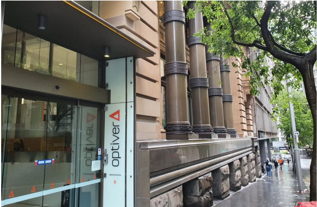
Figure 2-16 Heritage listed commercial building at 39 Hunter Street
