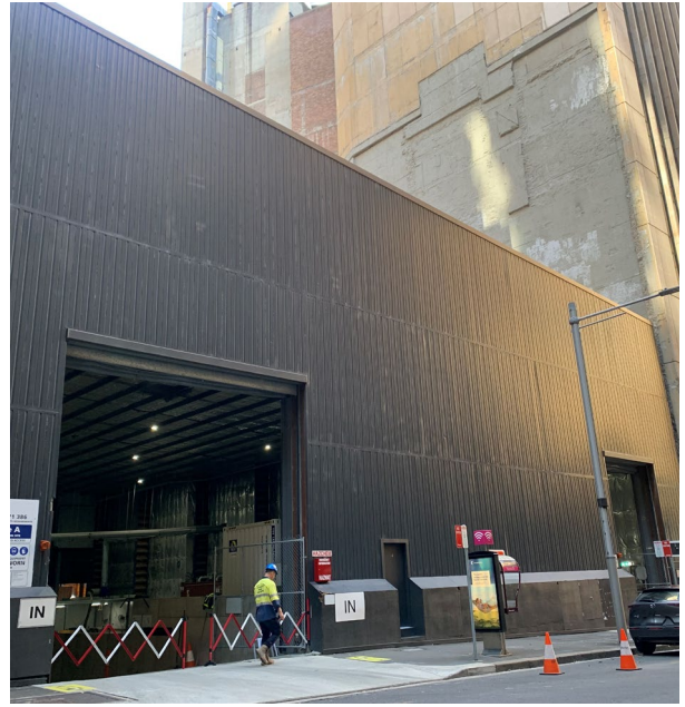
Figure 2-6 Construction site at 33 Blich Street and existing office building at 37 Blich Street
