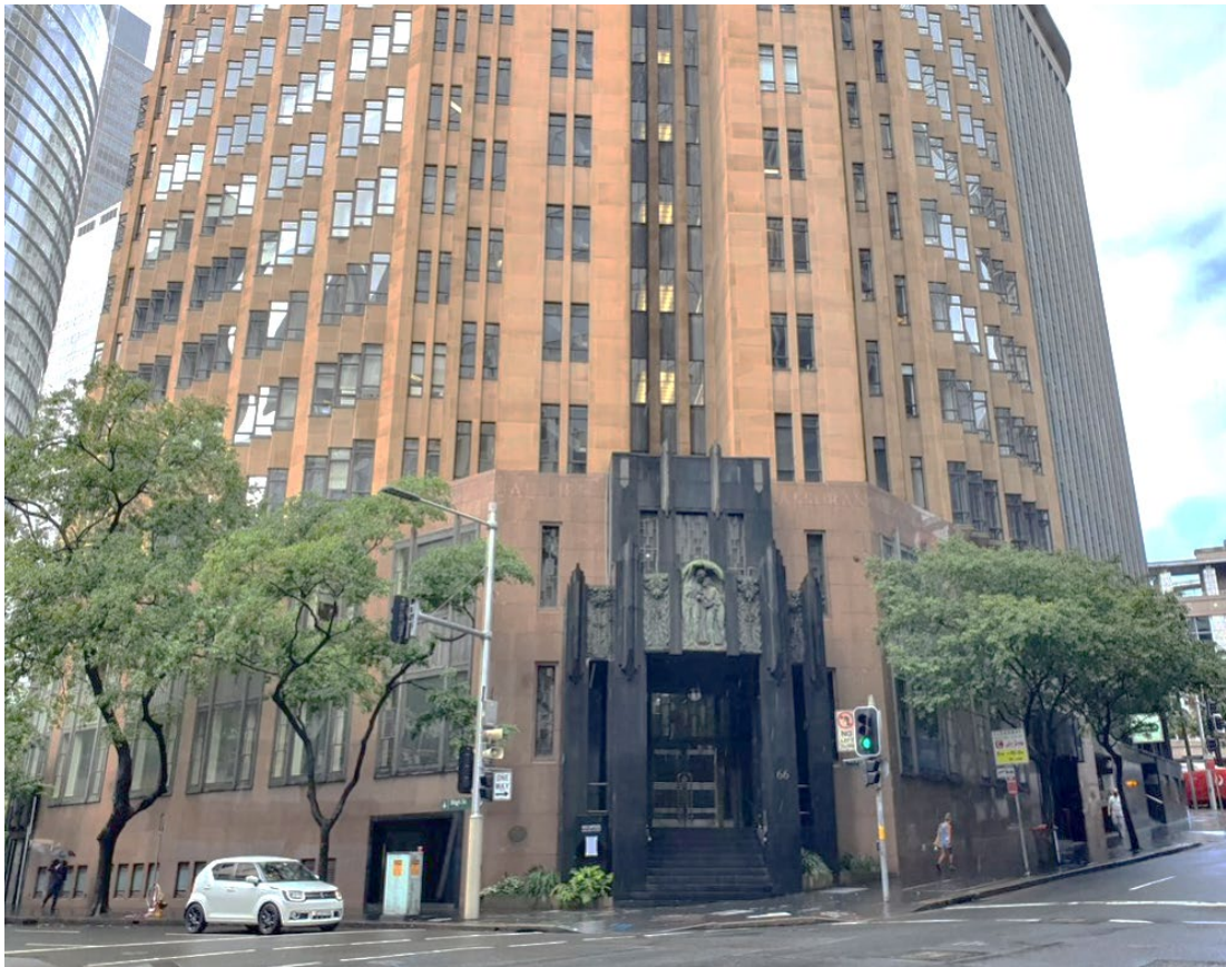
Figure 2-14 Heritage listed City Mutual Life Assurance Building at 10 Bligh Street
