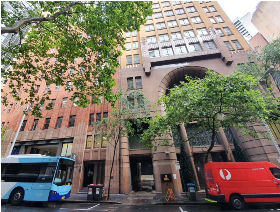
Figure 2-11 Existing heritage listed buildings at 12-14 and 16 O'Connell Street
