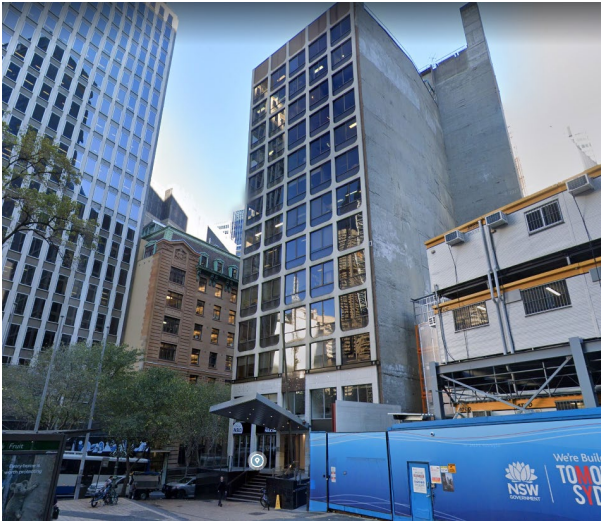
Figure 2-10 View of 48 Hunter Street, facing south west
