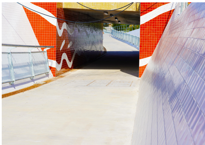
Nigel Love Bridge underpass.
