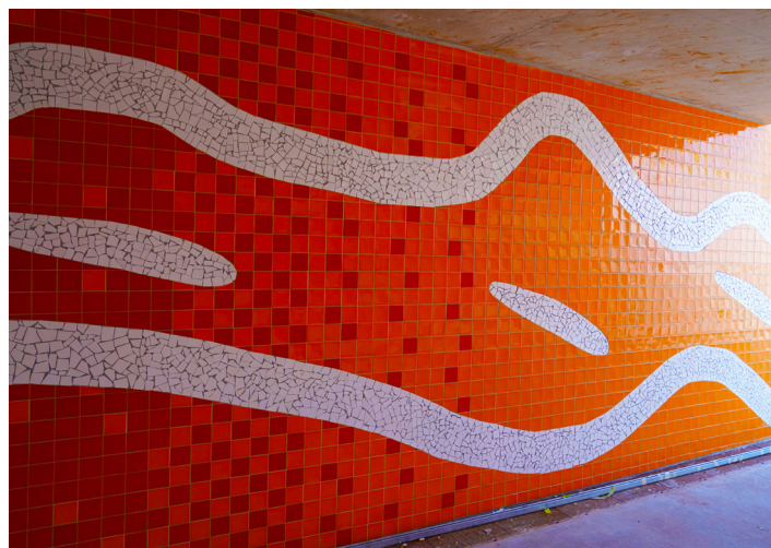
Nigel Love Bridge underpass users will note the ochre tiling.
