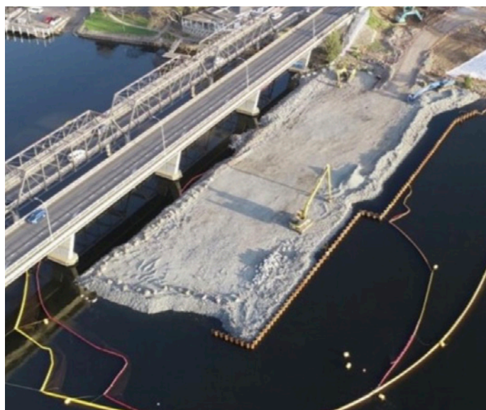
Example of rock platform construction (Nowra Bridge)
