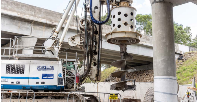
Piling activities at Villiers Road, Cecil Park
