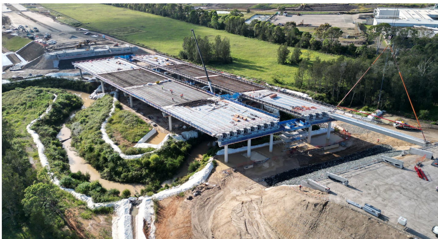
Lifting girders on Badgerys Creek bridge
