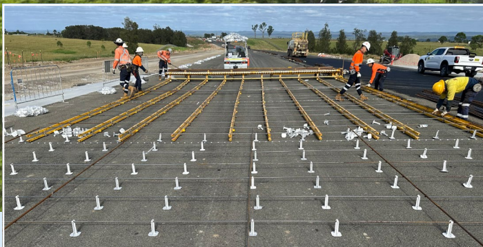
Installing steel reinforcement
