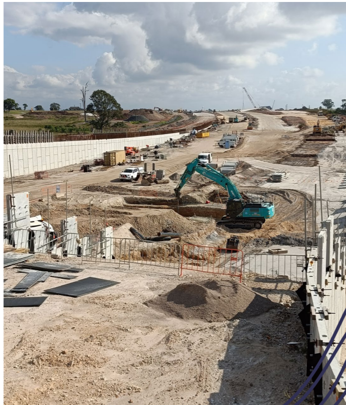
Building Airport Access Road looking north
