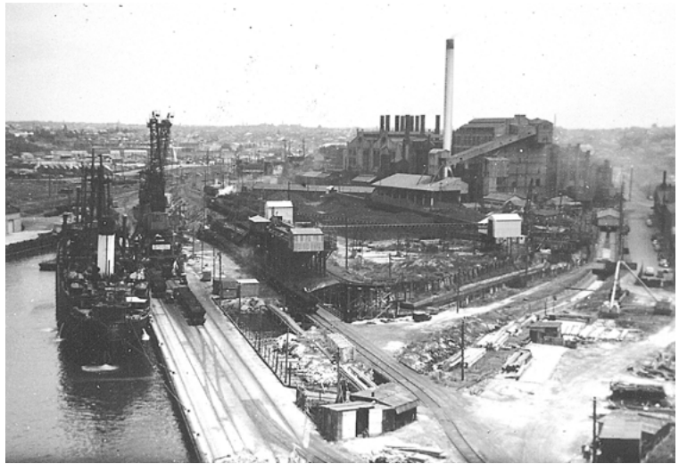
White Bay Power Station. Credit: City of Sydney Archives.
