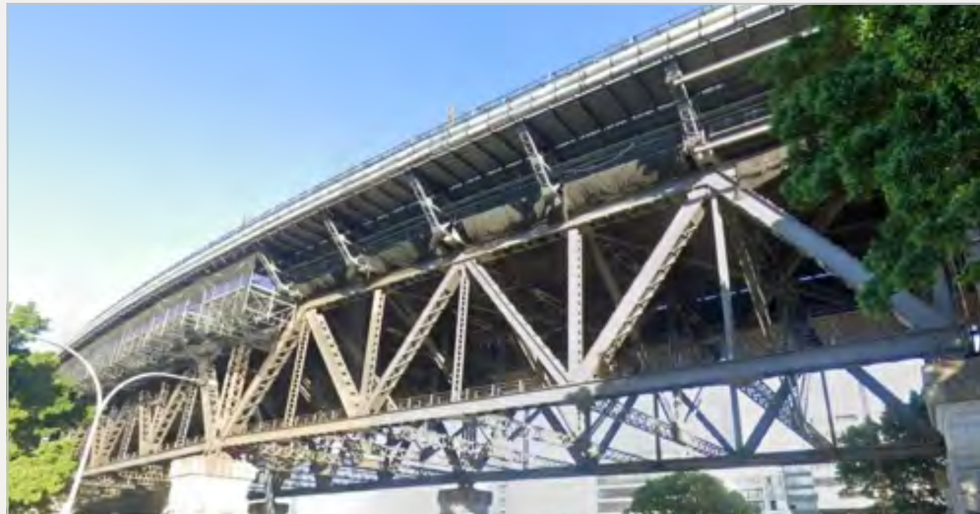
Figure B.19 Existing cantilevered footpath
