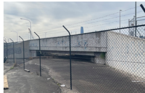
Figure 84: Robert Street culvert
