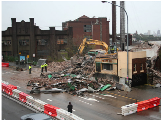
Figure 64: Demolition of White Bay Hotel after fire, 2008. Peter Fletcher
