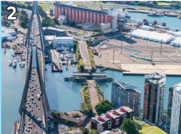
Figure 7: Glebe Island Bridge. Courtesy of DPE
