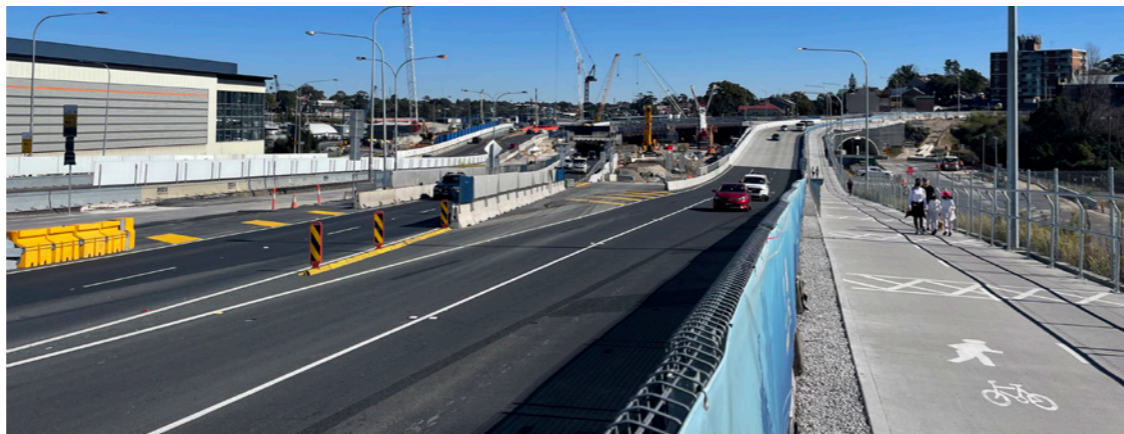
Figure 83: Construction of Rozelle Bay interchange with temporary shared active transport link
