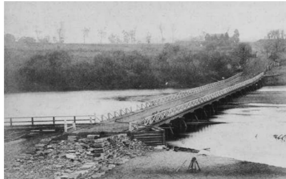
Figure 67: View west in 1871 from Glebe Island to a bridge about 100m in length spanning from Balmain to Glebe Island linking to Victoria Road to the north
