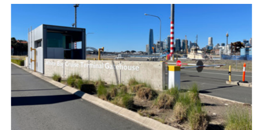
Figure 24: White Bay Cruise Terminal Gatehouse
