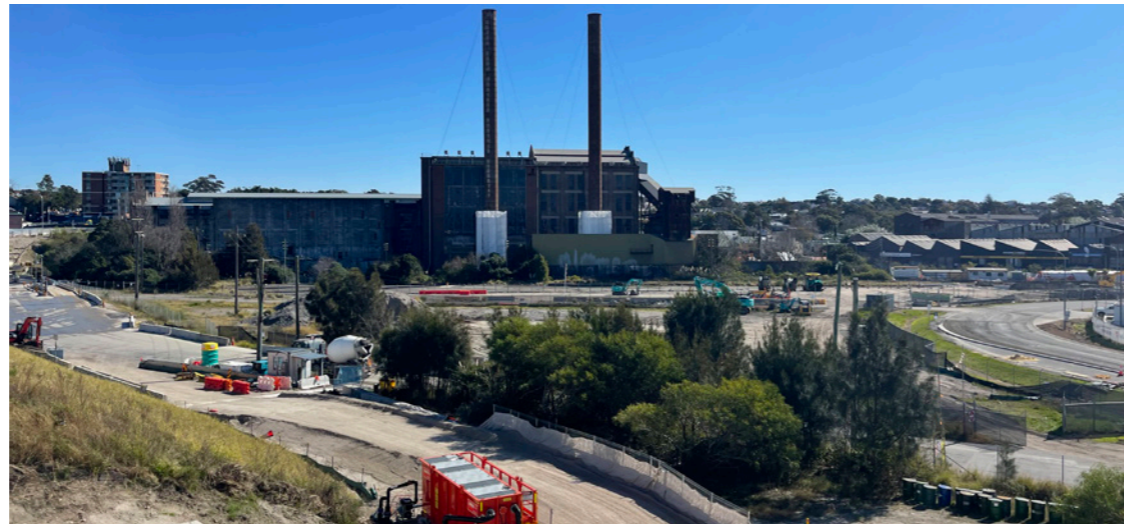
Figure 82: White Bay Sub-precinct with temporary works
