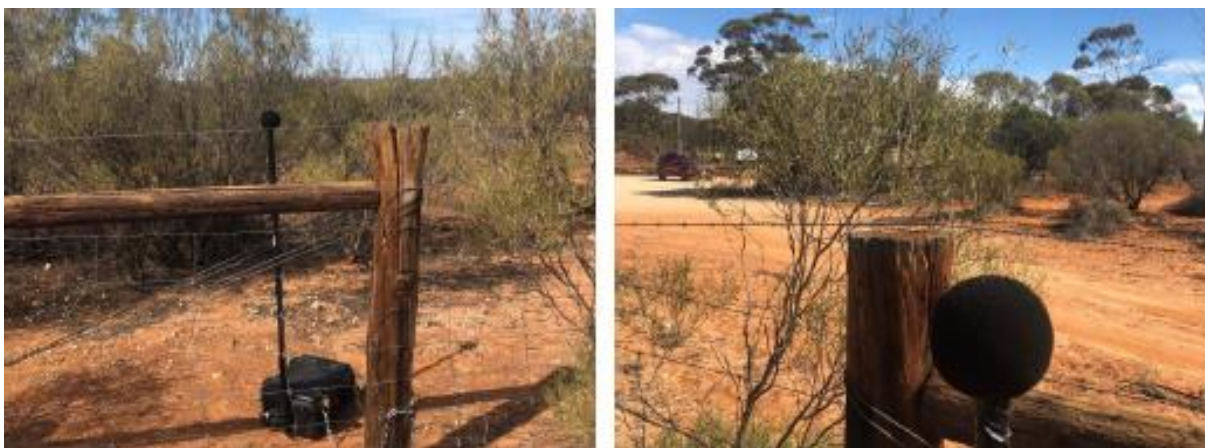
Plate 15-1: Noise logger installation
