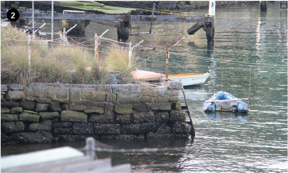
Figure 61: Existing seawalls in poor condition
