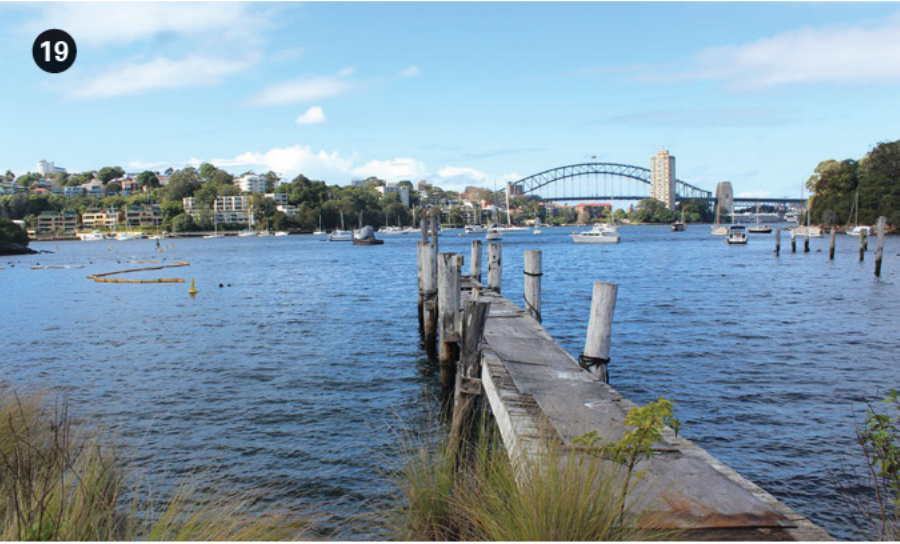
Figure 38: Derelict timber wharf
