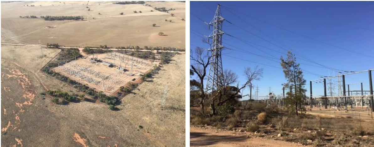
Plate 2-1: Existing Robertstown substation
