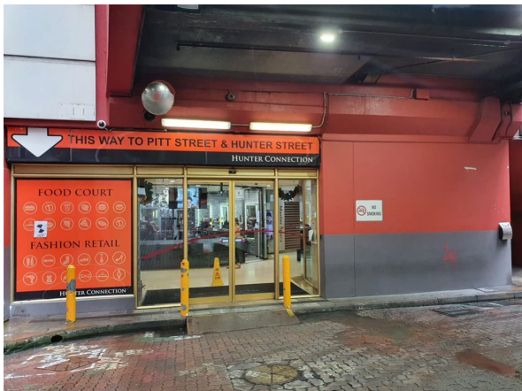
Figure 2-8 De Mestre Place with overpass above (5010 De Mestre Place)
