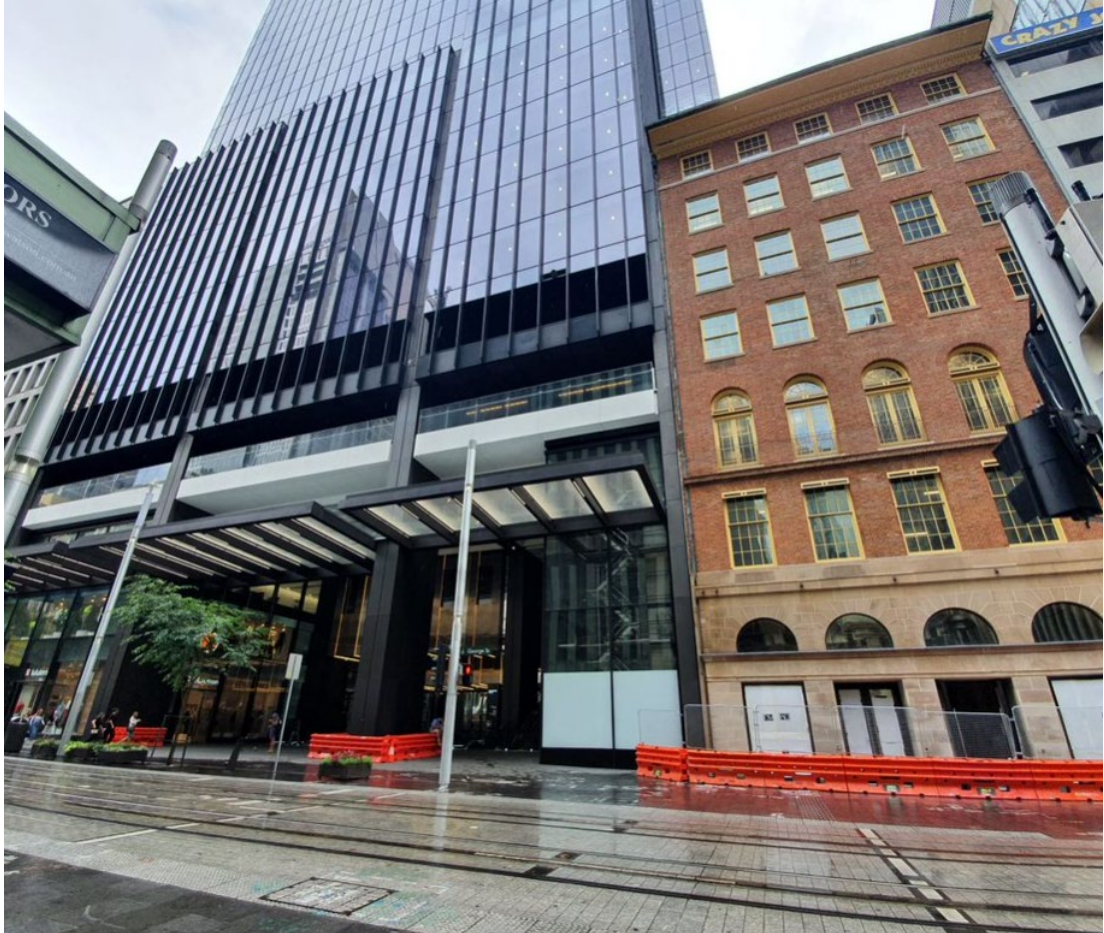
Figure 2-14 Brookfield Place and 285-287 George Street
