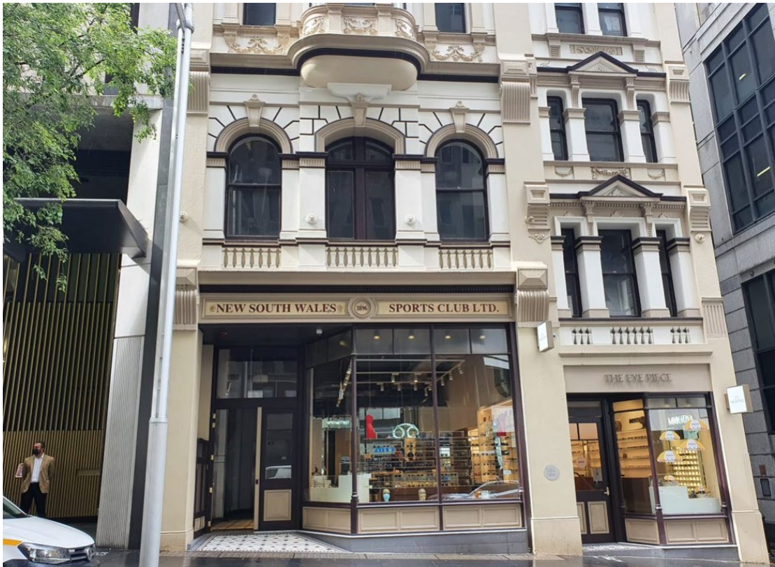
Figure 2-11 Commercial buildings on the opposite side of Hunter Street
