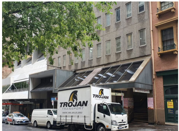
Figure 2-9 Existing commercial building at 5 Hunter Street
