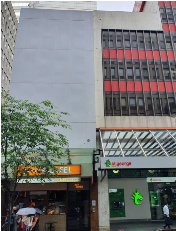
Figure 2-6 Existing commercial buildings at 312 and 314-318 George Street
