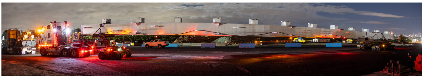
The first delivery for Sydney Gateway's twin arch bridges
