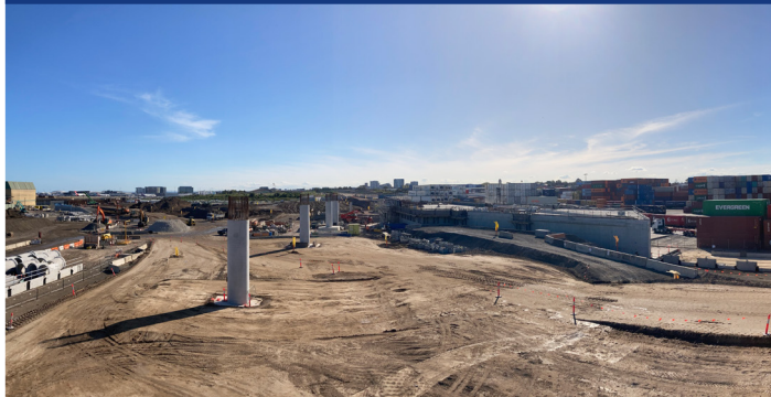
Bridge abutments taking shape at our St Peters site.
