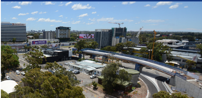
The flyover and ramp down Sir Reginald Ansett Drive heading towards the Domestic Terminals.
