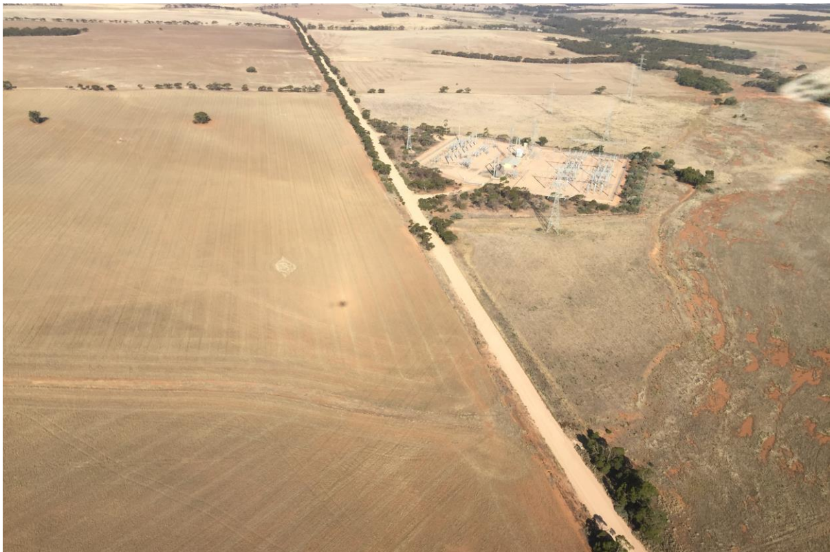
Plate 9-1: Robertstown substation and surrounding land uses (looking south-east)
