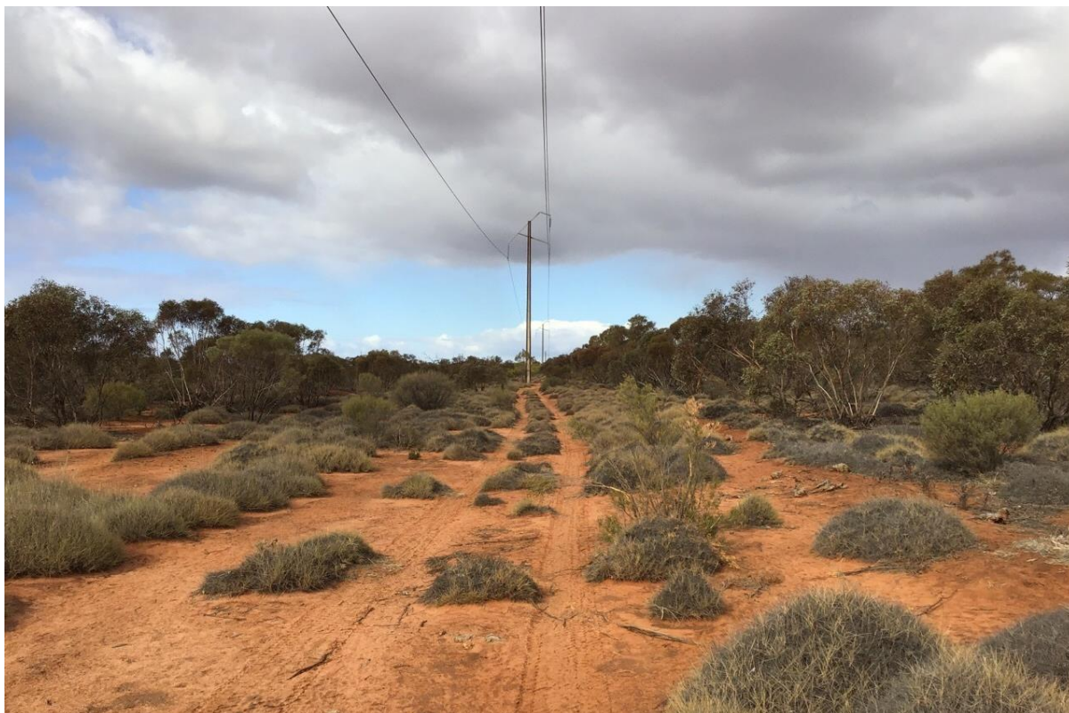
Plate 9-11: 132 kV line easement on Hawks Nest Station (looking south-east)
