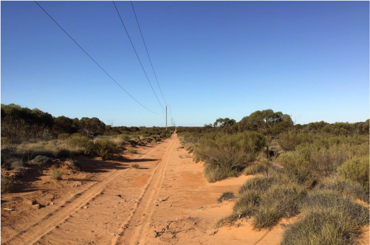
Plate 9-9: Existing transmission line on southern boundary of Taylorville Station
