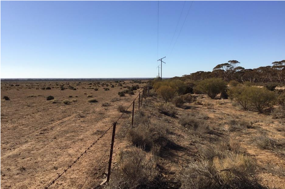
Plate 9-4: Existing transmission line along Powerline Road
