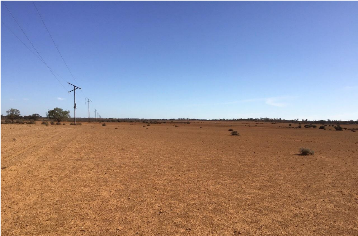
Plate 9-7: Existing transmission line traversing pastoral land north of boundary of White Dam Conservation Park (looking south-east)
