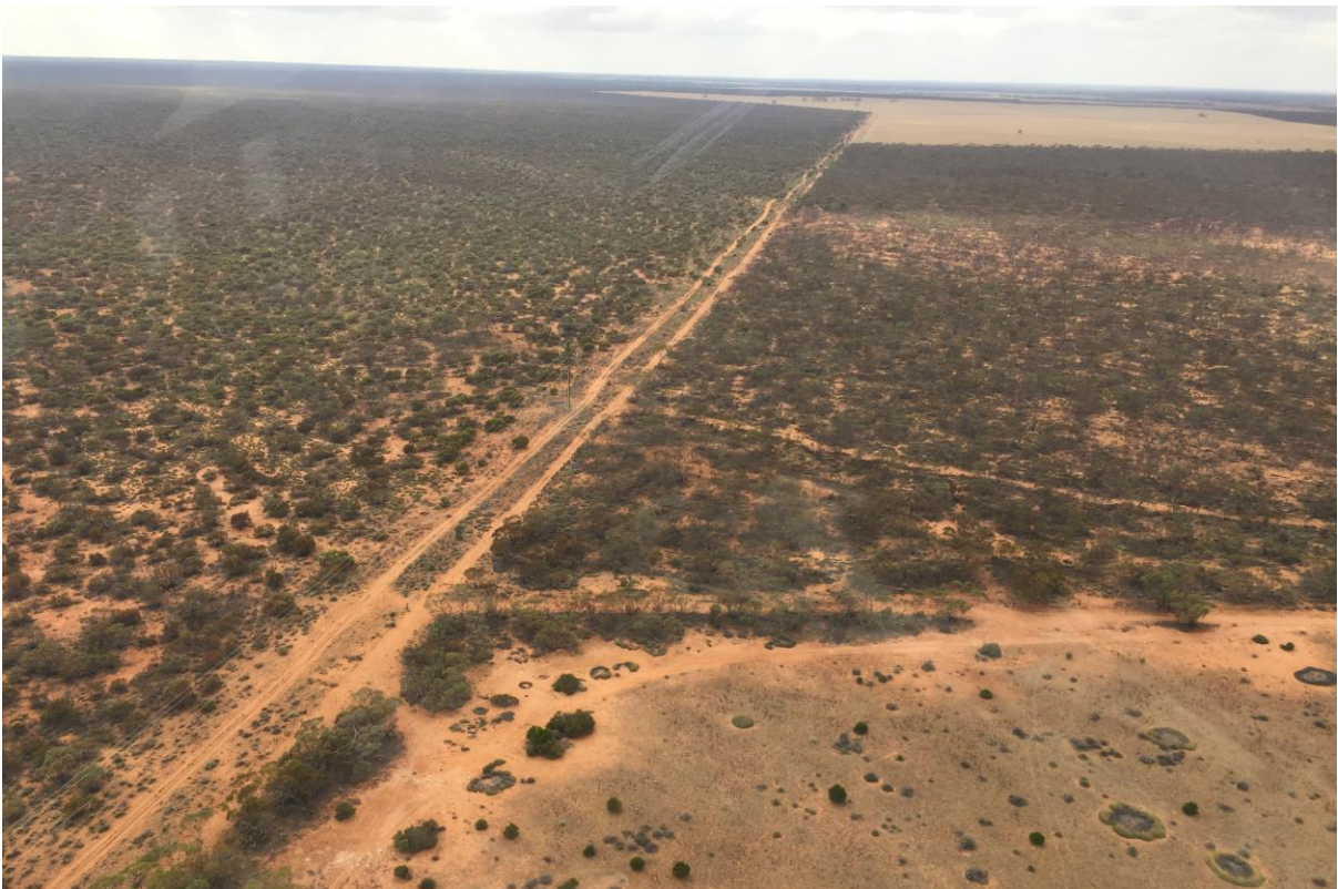
Plate 9-8: Existing transmission line and easement approximately 6 km west of Taylorville Station (looking south-east)
