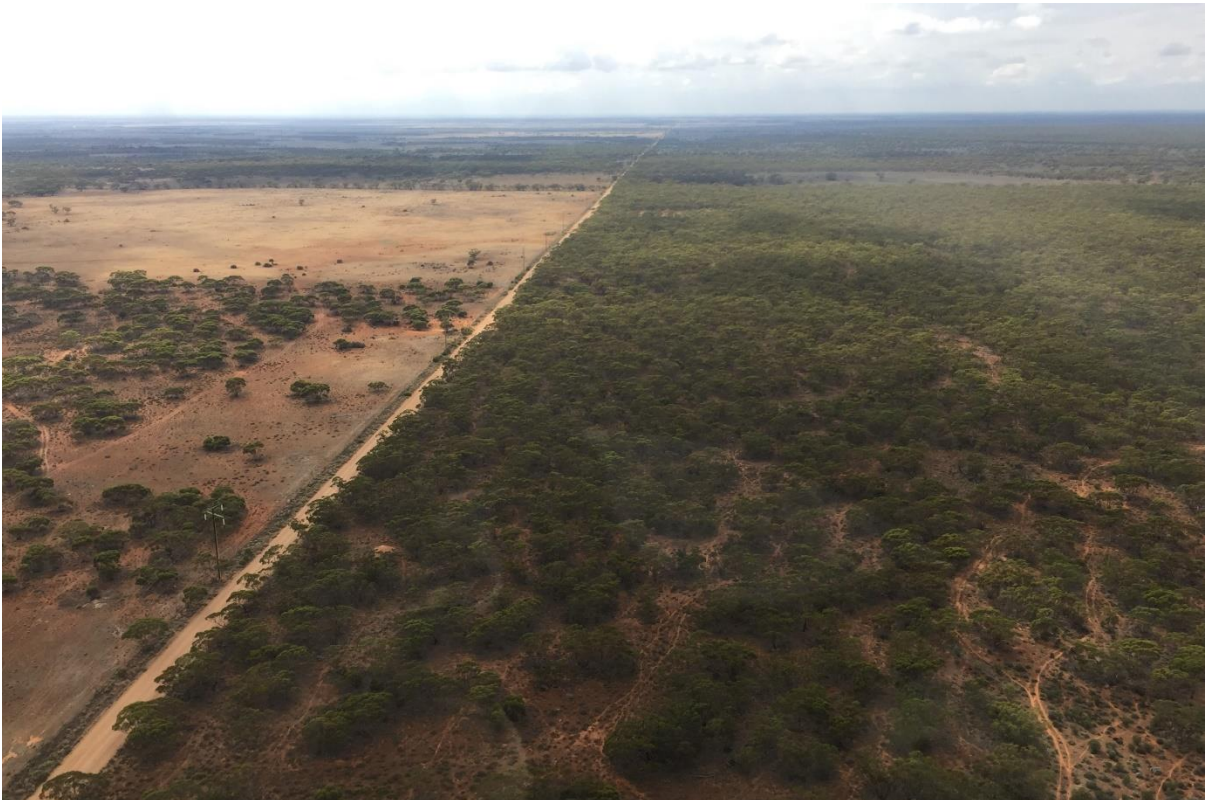
Plate 9-3: Powerline Road and existing ElectraNet transmission line (132 kV) (looking east)
