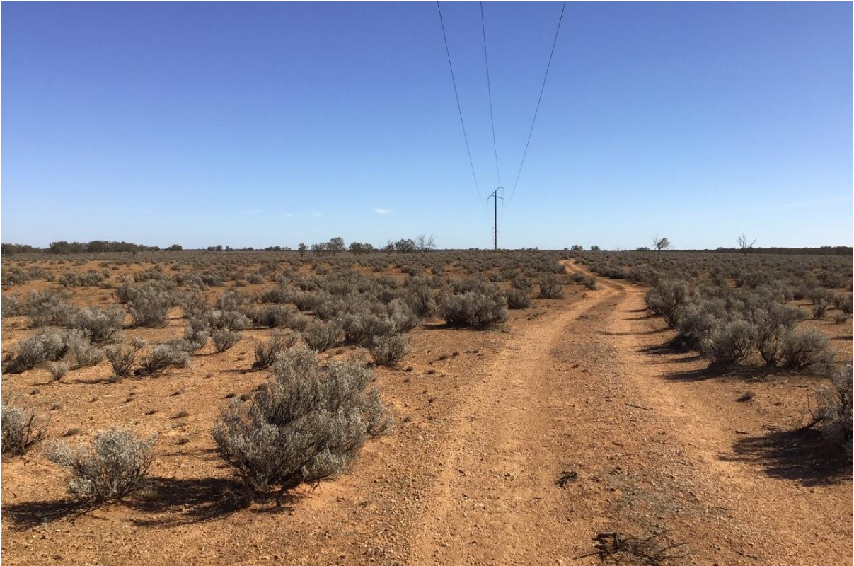
Plate 9-5: Existing track and transmission line within the White Dam Conservation Park west of crossing of Goyder Highway
