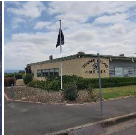
Figure 236: Windsor Country Golf Clubhouse (Source: Google Maps, 2022)
