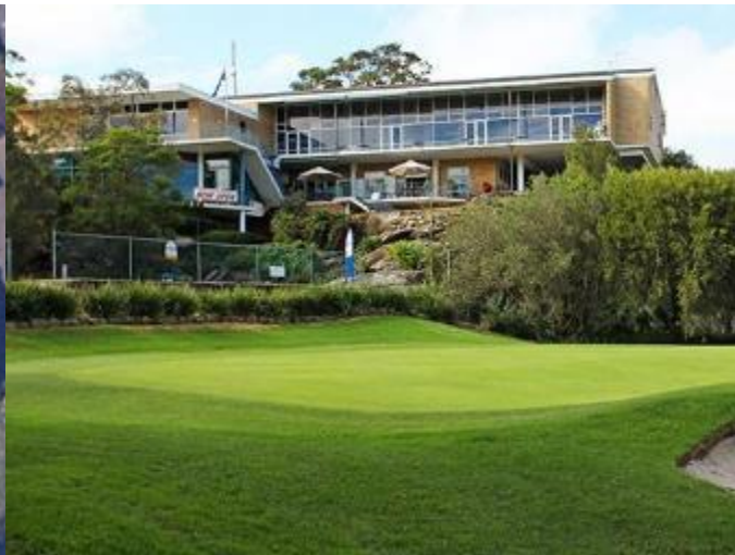
Figure 61: Castlecove Golf Clubhouse (Source: Golf Course Solutions, 2022)
