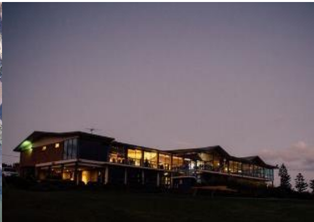
Figure 136: Mona Vale Golf Clubhouse (Source: Mona Vale Golf Club, 2022)
