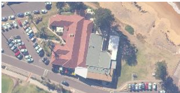
Figure 116: Aerial of Long Reef Golf Clubhouse (Source: Six Maps, 2022)
