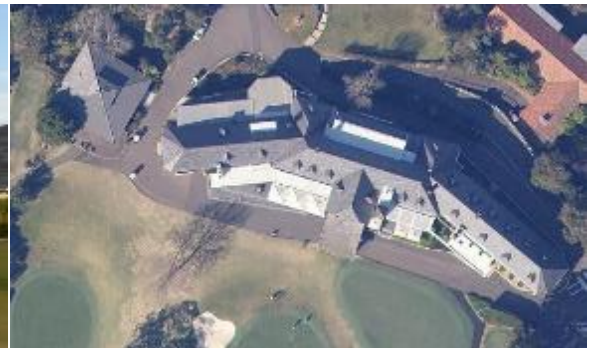
Figure 90: Aerial photograph of Elanora Golf Course Clubhouse (Source: Six Maps, 2022)
