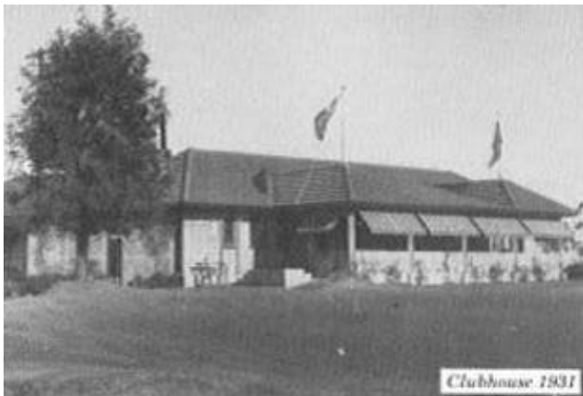
Figure 168: Photograph of the Clubhouse in 1931 (Source: Oatlands Golf Club)
