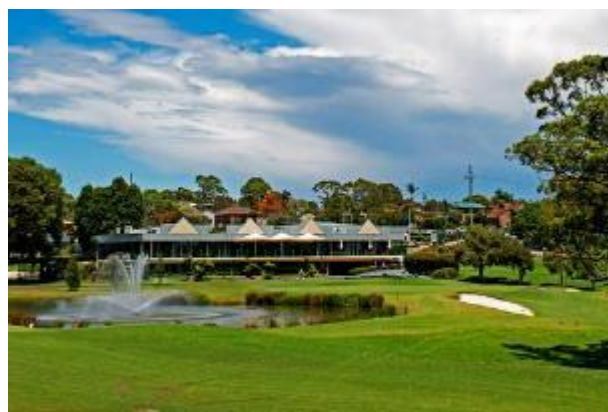
Figure 153: North Ryde Clubhouse (Source: Golfer.com, 2022)
