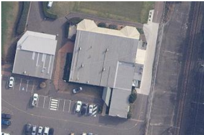
Figure 235: Aerial of Windsor Country Golf Clubhouse (Source: Six Maps, 2022)
