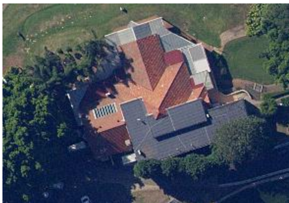
Figure 50: Aerial of Cammeray Golf Clubhouse (Source: Six Maps, 2022)
