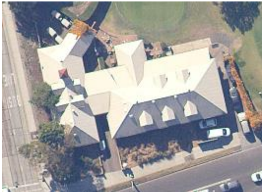
Figure 229: Aerial of Warringah Golf Clubhouse (Source: Six Maps, 2022)
