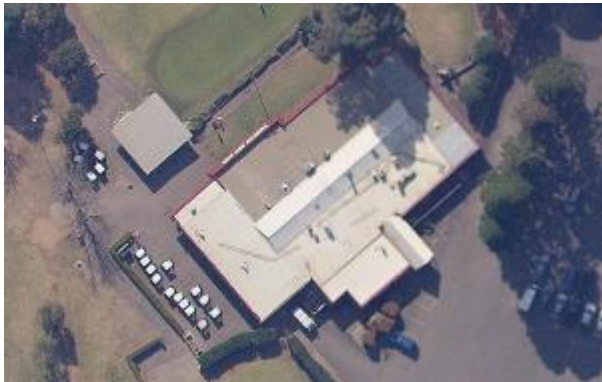
Figure 84: Aerial of Dunheved Golf Clubhouse (Source: Six Maps, 2022)
