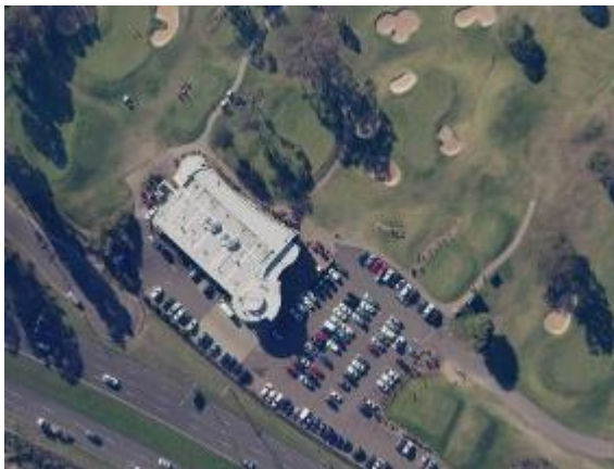
Figure 94: Aerial of Fox Hills Golf Clubhouse (Source: Six Maps, 2022)
