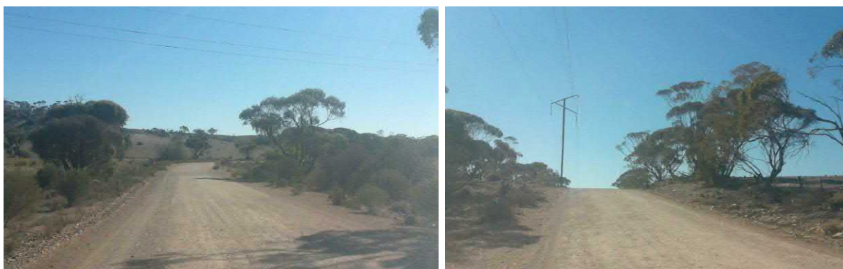
Figure 5 Section of Powerline Road with poor delineation, particularly around curves (left) and an unsigned crest (right)
