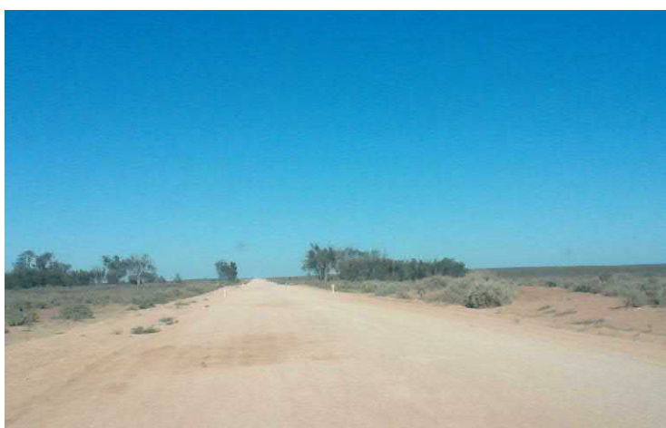
Figure 9 Example of failed pavement along Wentworth Renmark Road
