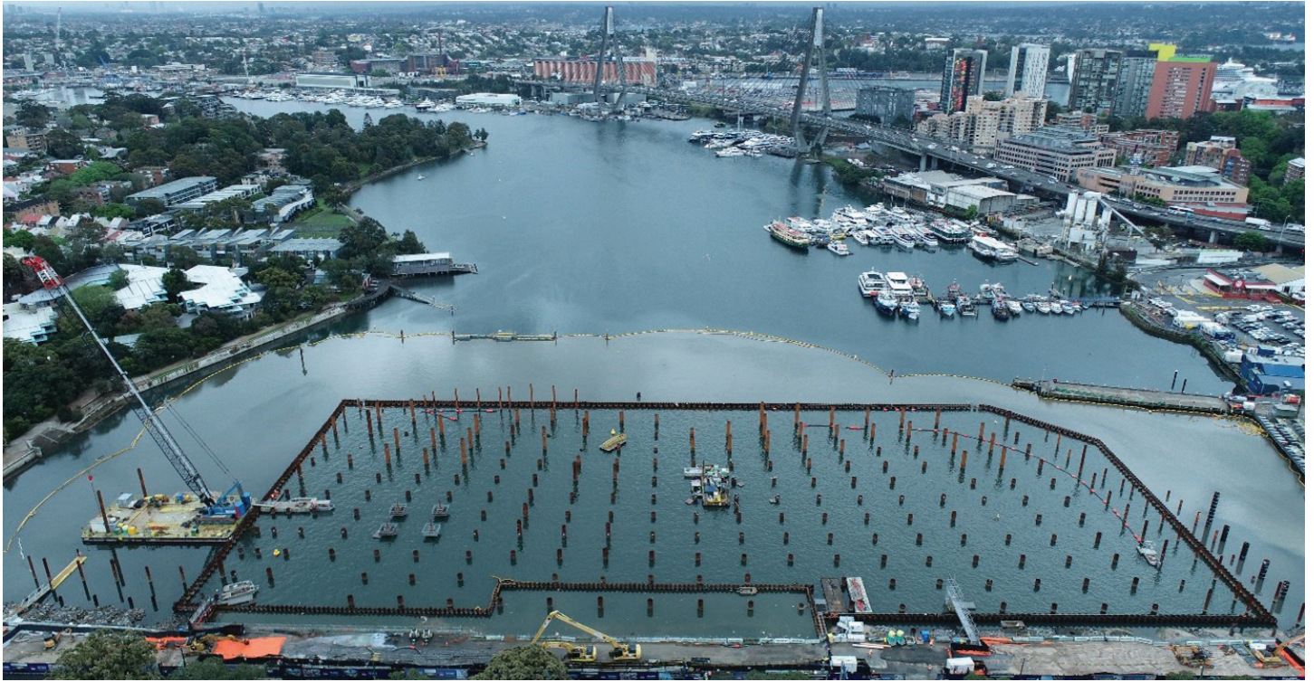
^ The new Sydney Fish Market construction site – looking north
