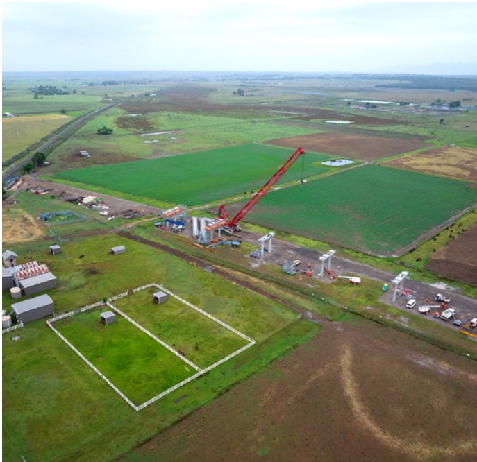
Bridge pier work on Doughboy Hollow looking east
