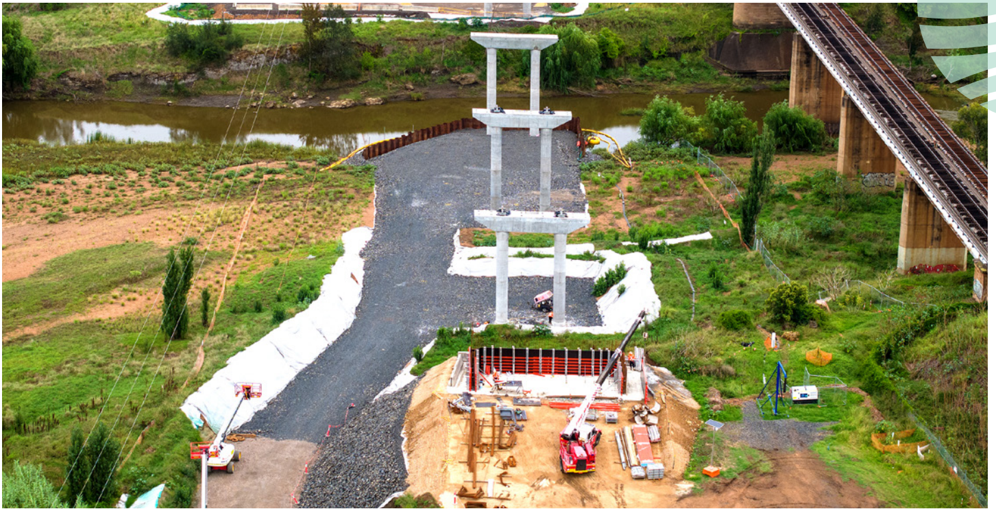
Bridge pier work at the Hunter River, looking north
