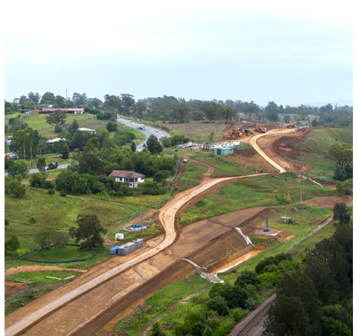
Earthworks at McDougalls Hill, looking north
