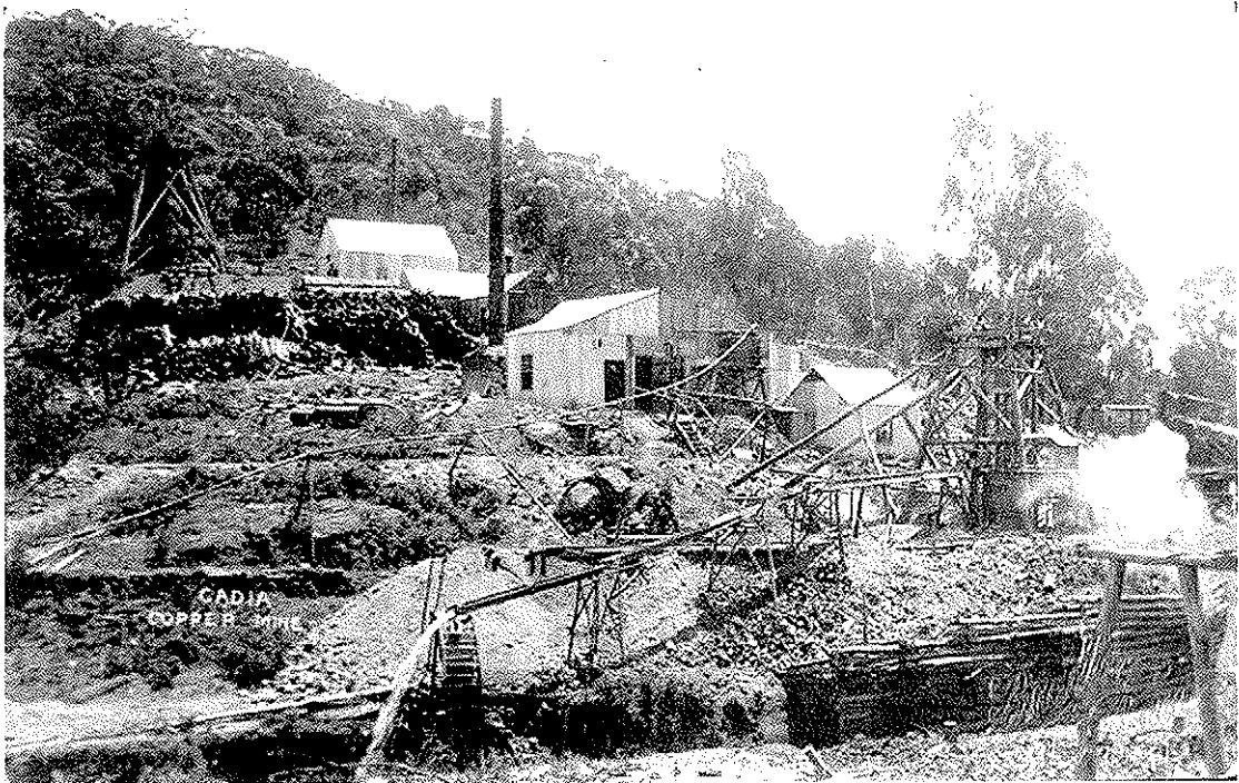
Cadia copper mine, State Library of NSW, looking west, note engine house, dewatering and water wheel
