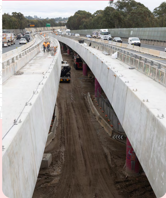
Concrete pour to join the new bridge deck to the existing bridge deck
