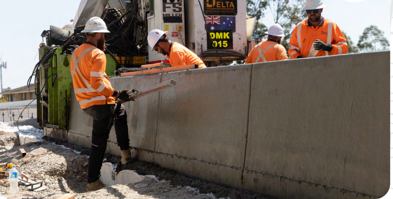
Barrier installation at the Elizabeth Drive Connection
