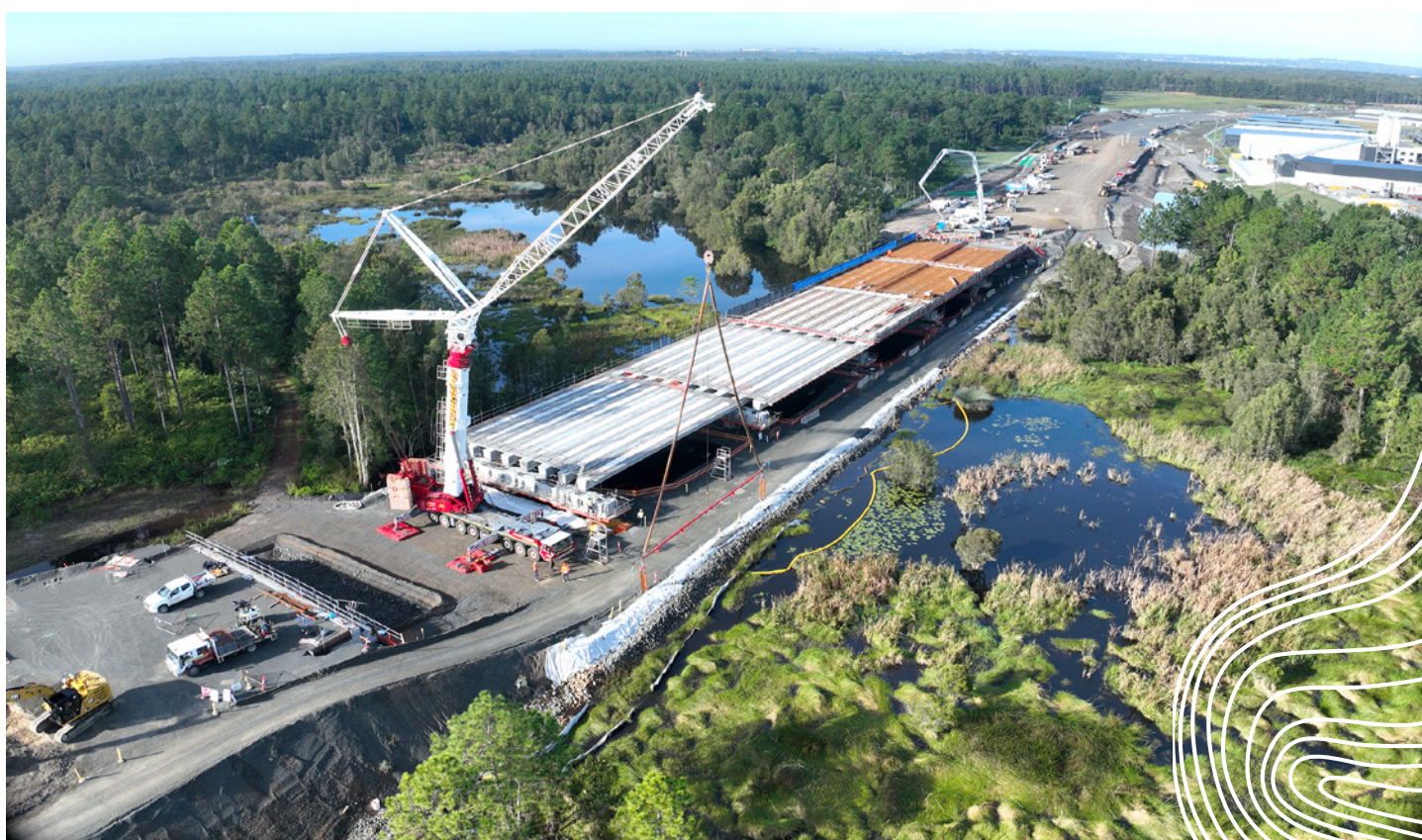
Girder installation at Windeyers Creek bridge
