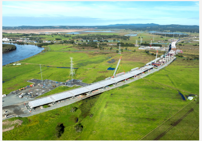
Viaduct construction progress at Tarro
