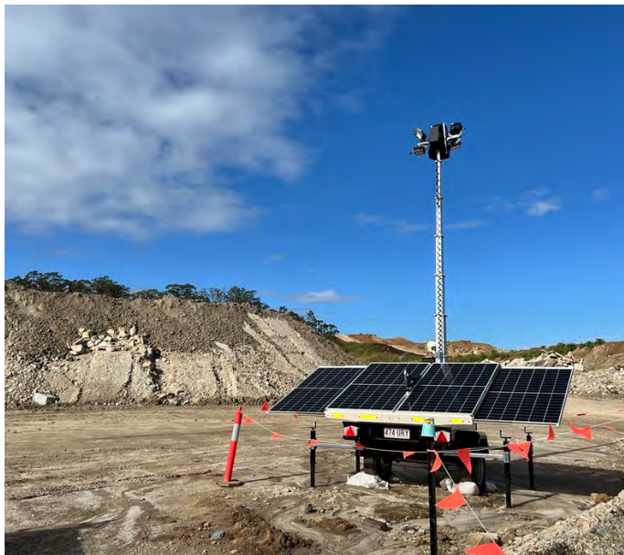
Figure 1: Solar light tower by stockpile area at AF9 compound.
