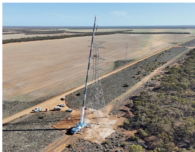
Image: Example of a 500kV transmission tower being assembled onsite from the EnergyConnect (NSW) project.
