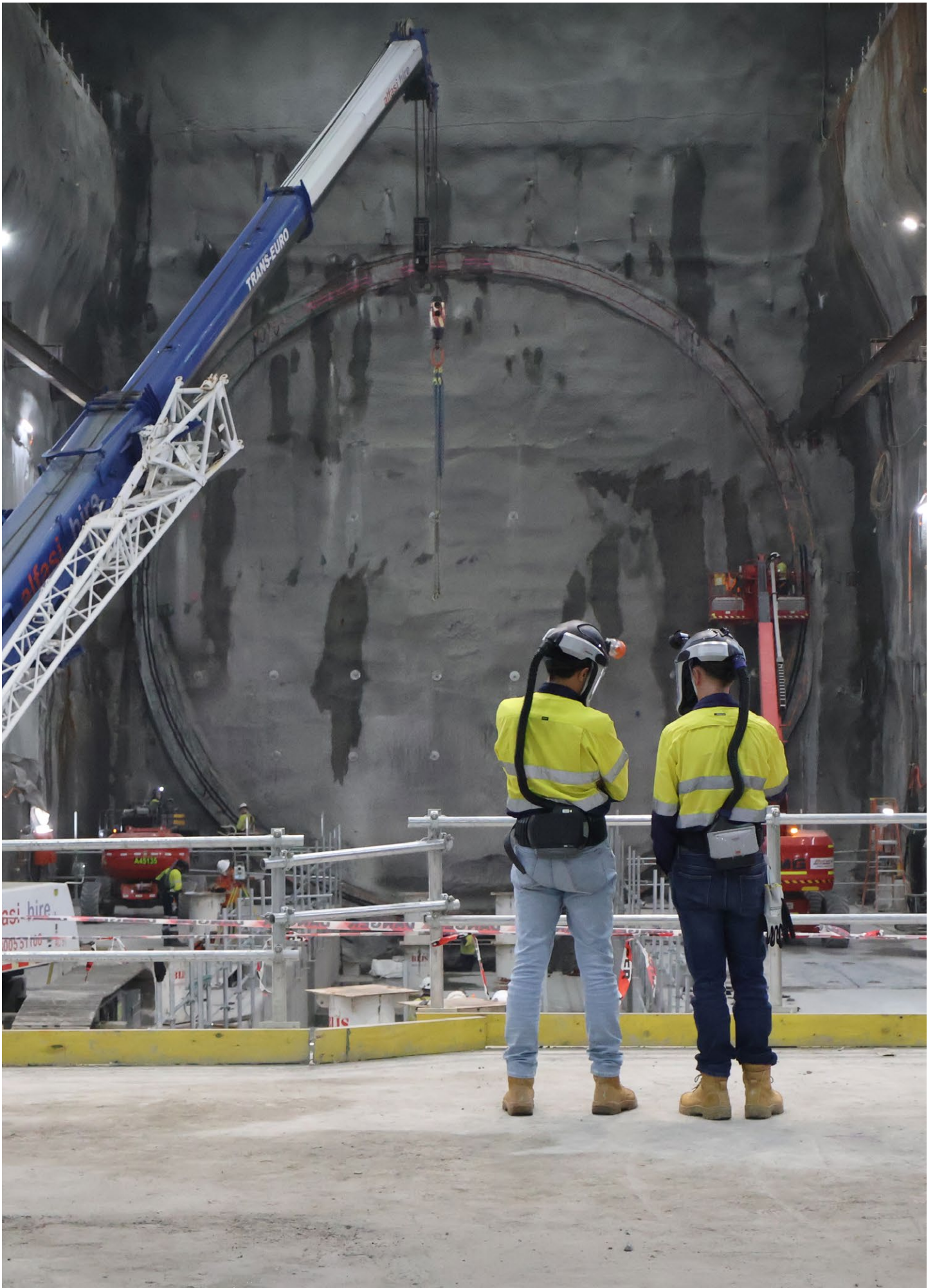
The TBM launch chambers under Birchgrove completed in November 2025.
