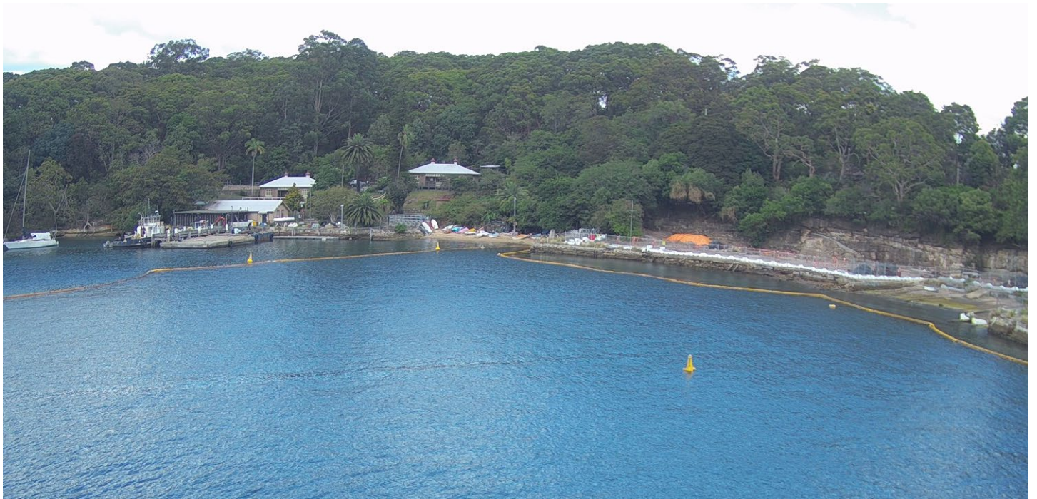
Derelict and hazardous maritime infrastructure in Berrys Bay now removed. (Looking west at the bay, now clear of hazards).
