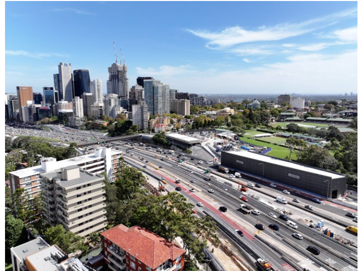
View south over the Warringah Freeway.
