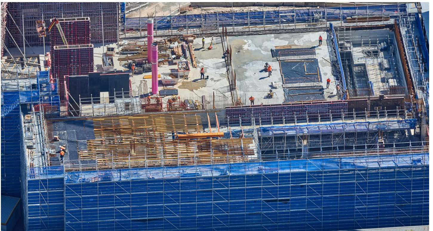
Construction progress - aerial view of the ventilation building, September 2025.
