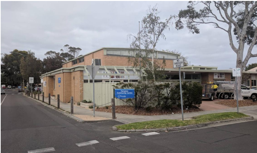
Photo: Outside Hampton Community Centre
