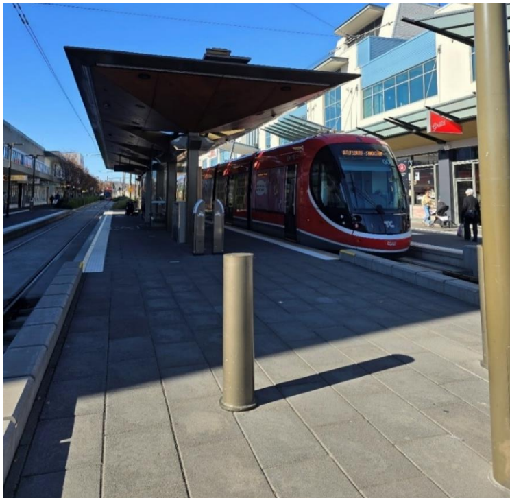
Figure 5-27 Example of an island platform arrangement, at the existing Gungahlin Place Stop
