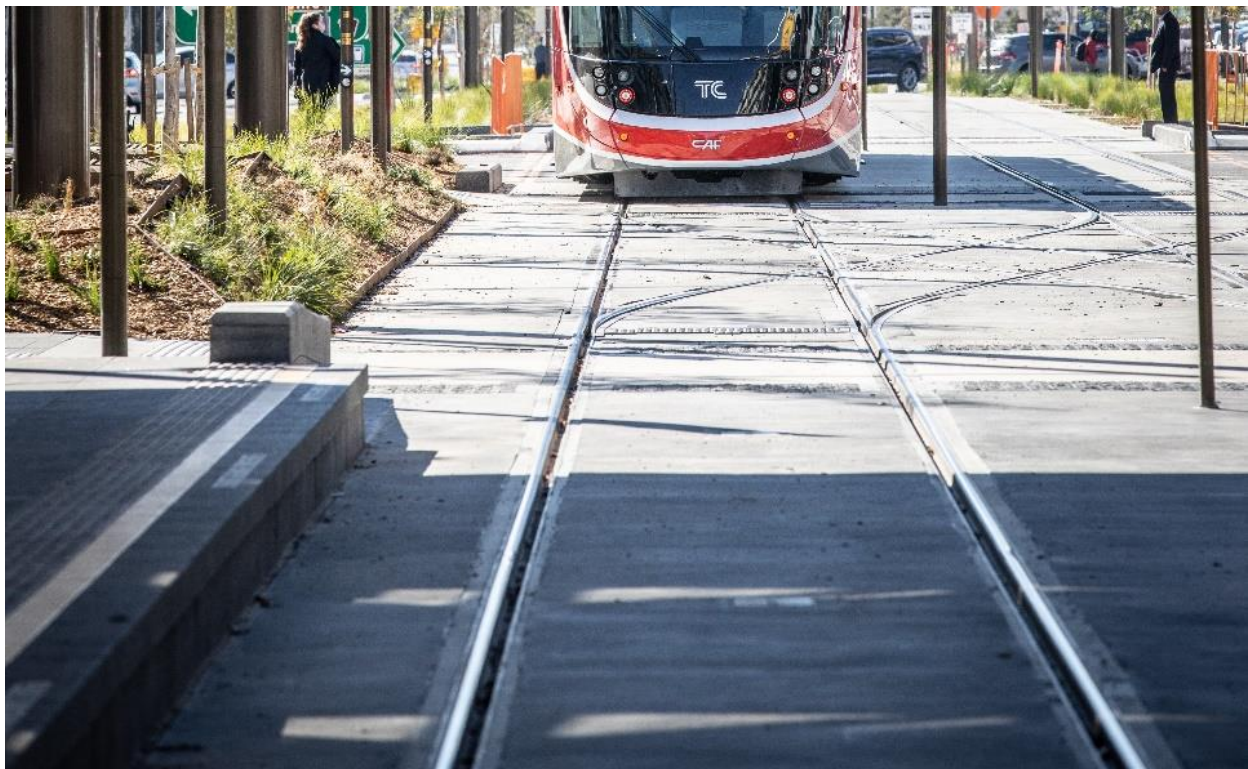
Figure 5-18 Image showing embedded tracks installed as part of LRS1
