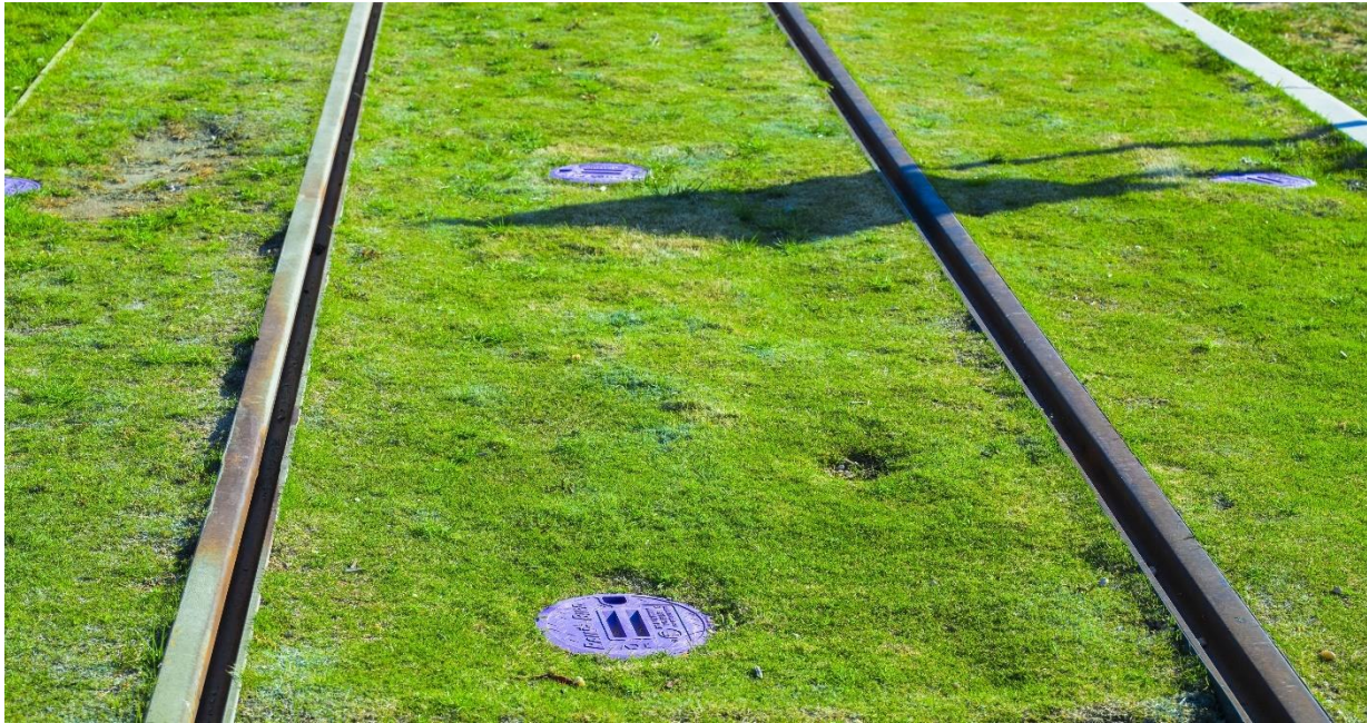
Figure 5-20 Example of green track – turf grass, from the light rail green track prototype at the National Arboretum Canberra (September 2024)
