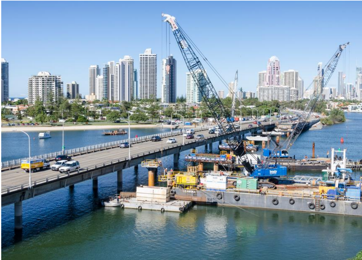
Figure 6-6 Example of a barge with a crane used in bridge construction works (Sundale Bridge Queensland, 2012-2014)
