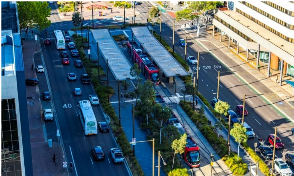
Figure 5-26 Example of a side platform arrangement at the existing Alinga Street Stop
