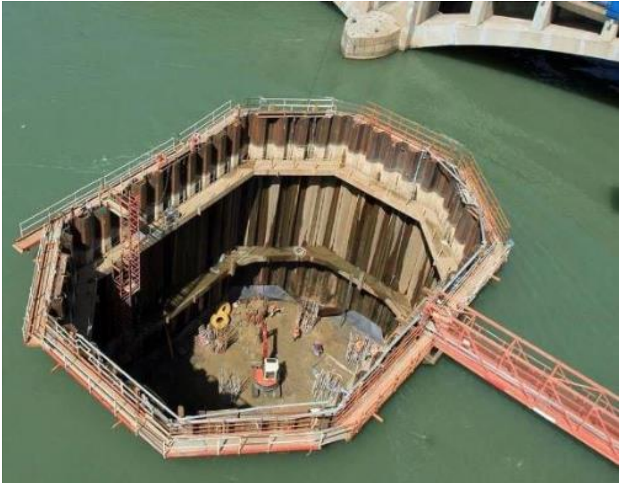
Figure 6-7 Example of a cofferdam structure (ED Corporation, 2024)
