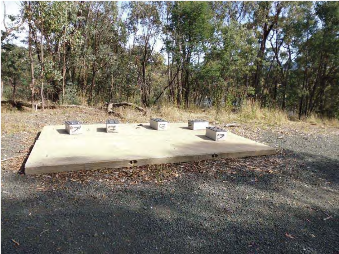
Photo 2 – Batteries stored in the open unbanded and not under cover.
