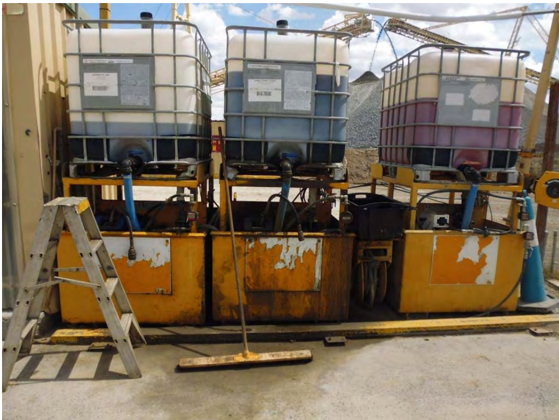
Photo 9 – IBCs stored in the open above metal bunds that can fill with water during rainfall.
