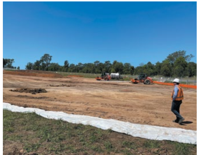
Construction of the new Wylde Mountain Bike Trail is underway
