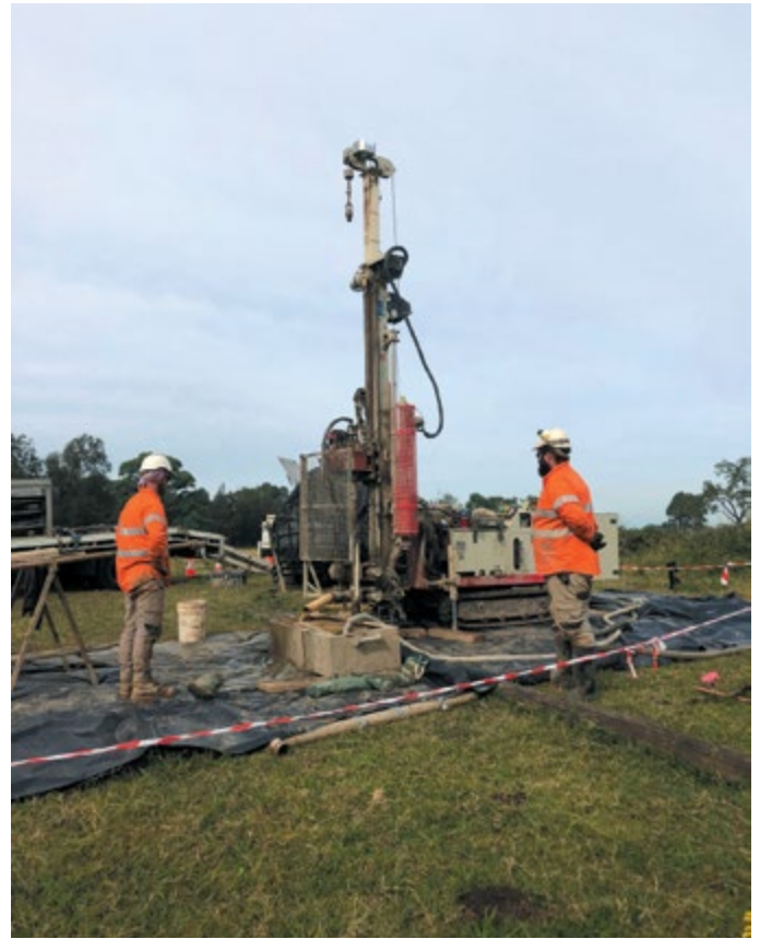
Geotechnical investigations near South Creek
